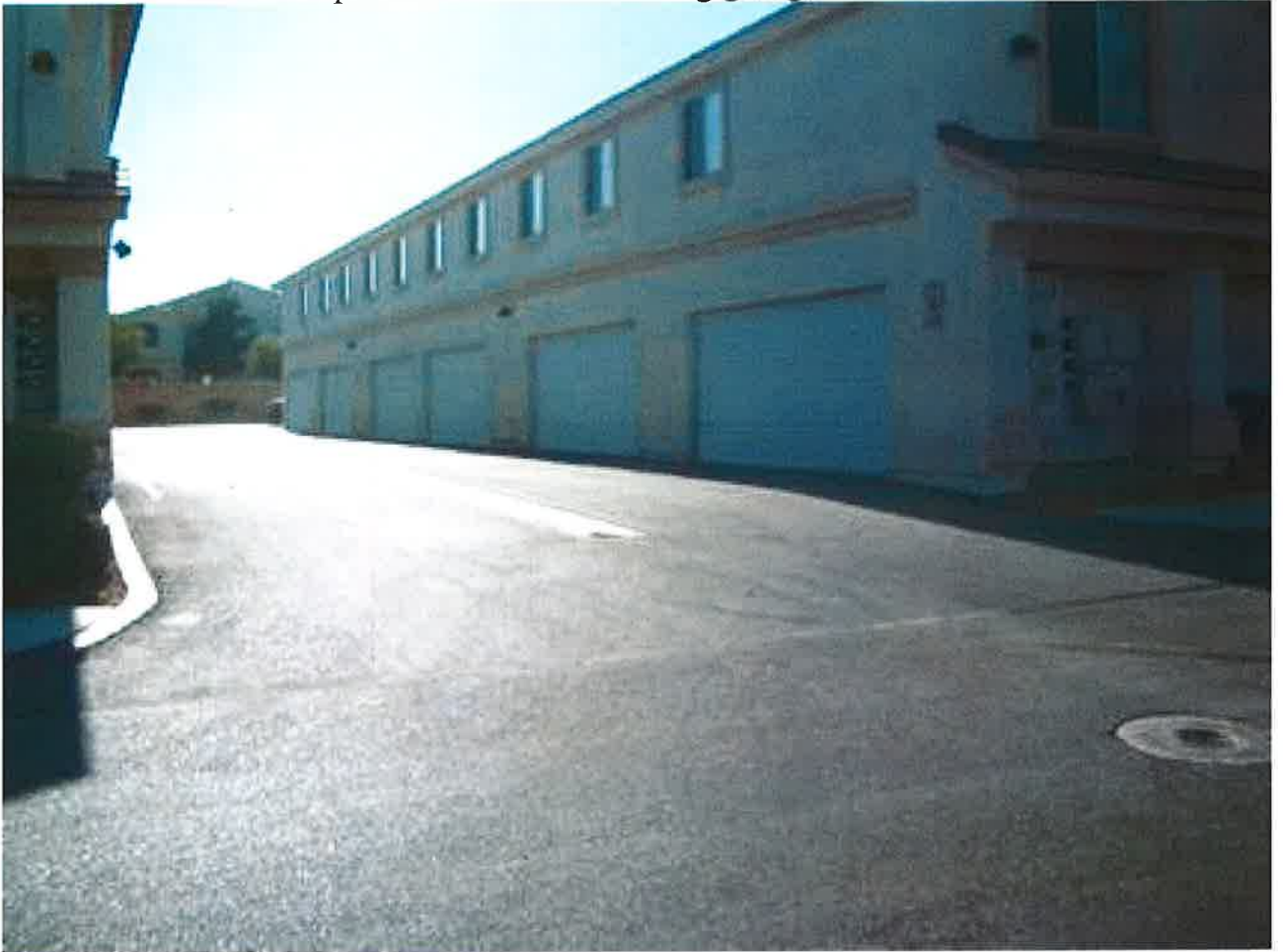
Rear of Apartment Homes showing garage entrance
