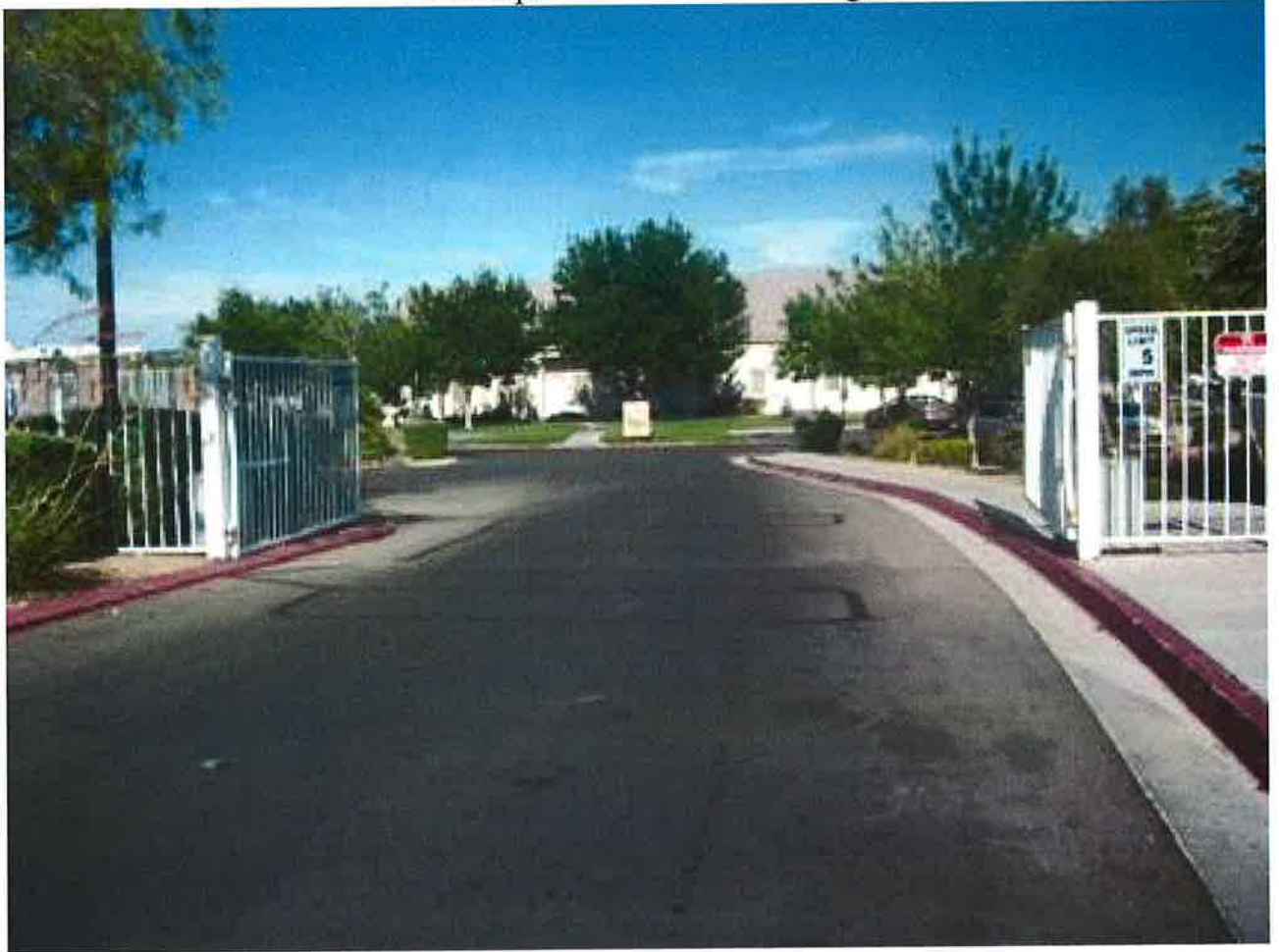
Entrance to Development with electronic gate
