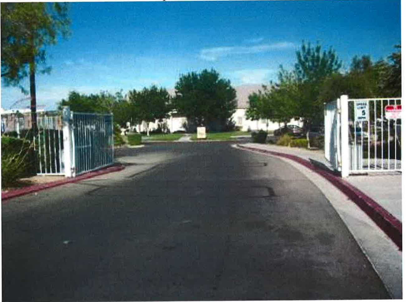
Entrance to Development with electronic gate
