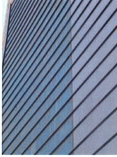
Metal Roofing with Firestone "Sierra Tan SR"
