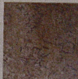
Toilet Room Wall Tile
