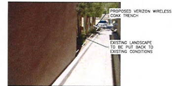
VIEW OF PROPOSED CONDUIT ROUTE (LOOKING NORTHEAST)
