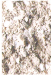
PERIMETER WALL MASONRY (FIELD)
