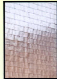
Typical Aluminum Metal Siding
