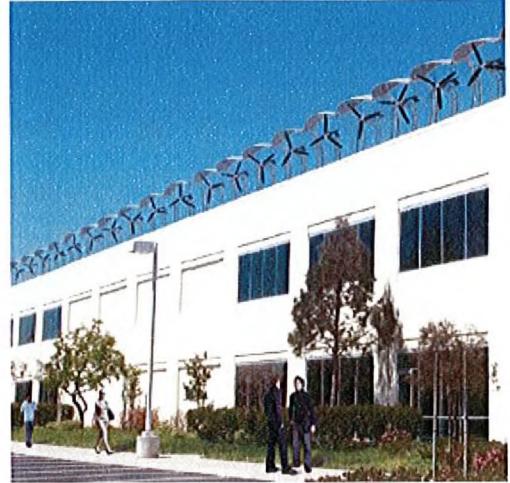
Roof-mounted horizontal axis system Manufacturer: AeroVironment Location: California
