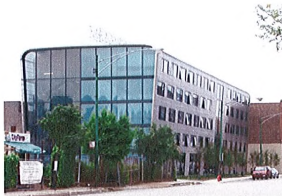
Roof-mounted horizontal axis system Manufacturer: Aerotecture International Location: Chicago, Illinois
