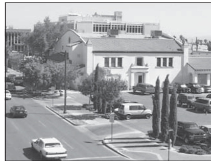
PHOTO 8: FOURTH STREET CORRIDOR IMPROVEMENTS
