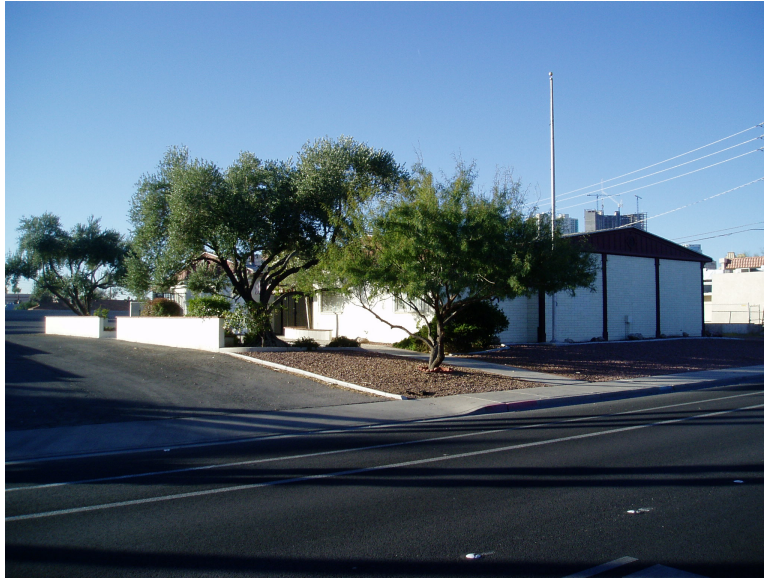
Front (north) and entrance (east) facades, looking southwest.
