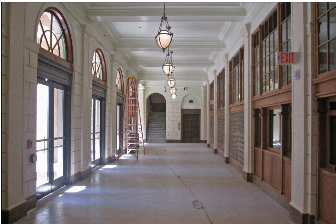
Photograph 22: Lobby, view west
