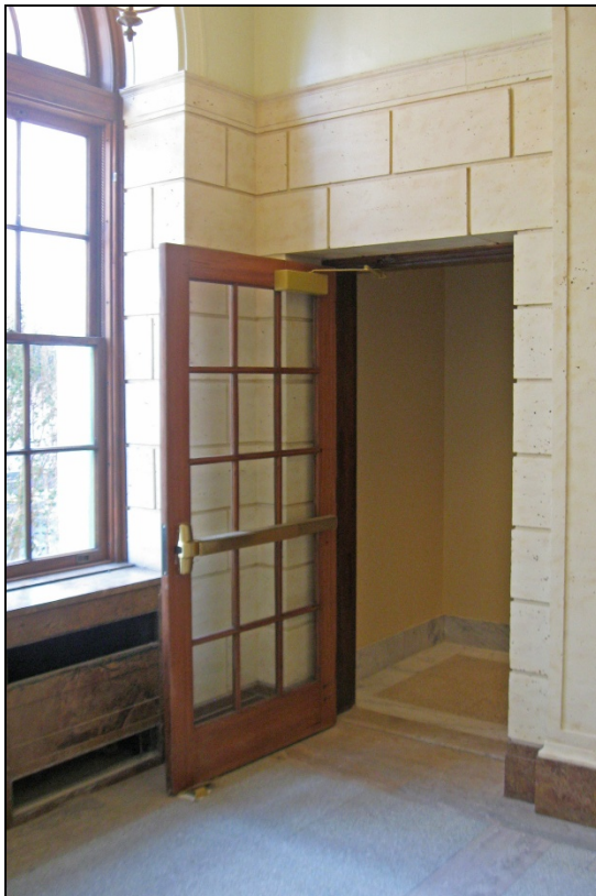
Photograph 26: Stair 1 door in lobby to basement, view southwest
