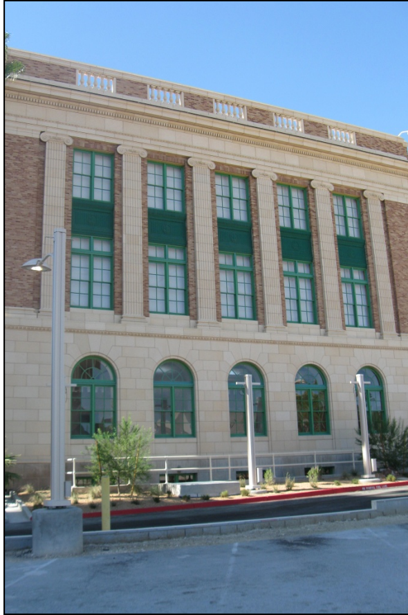
Photograph 3: West elevation, view west
