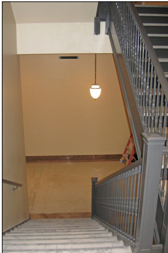
Photograph 42: Stair 1 at second floor, view west
