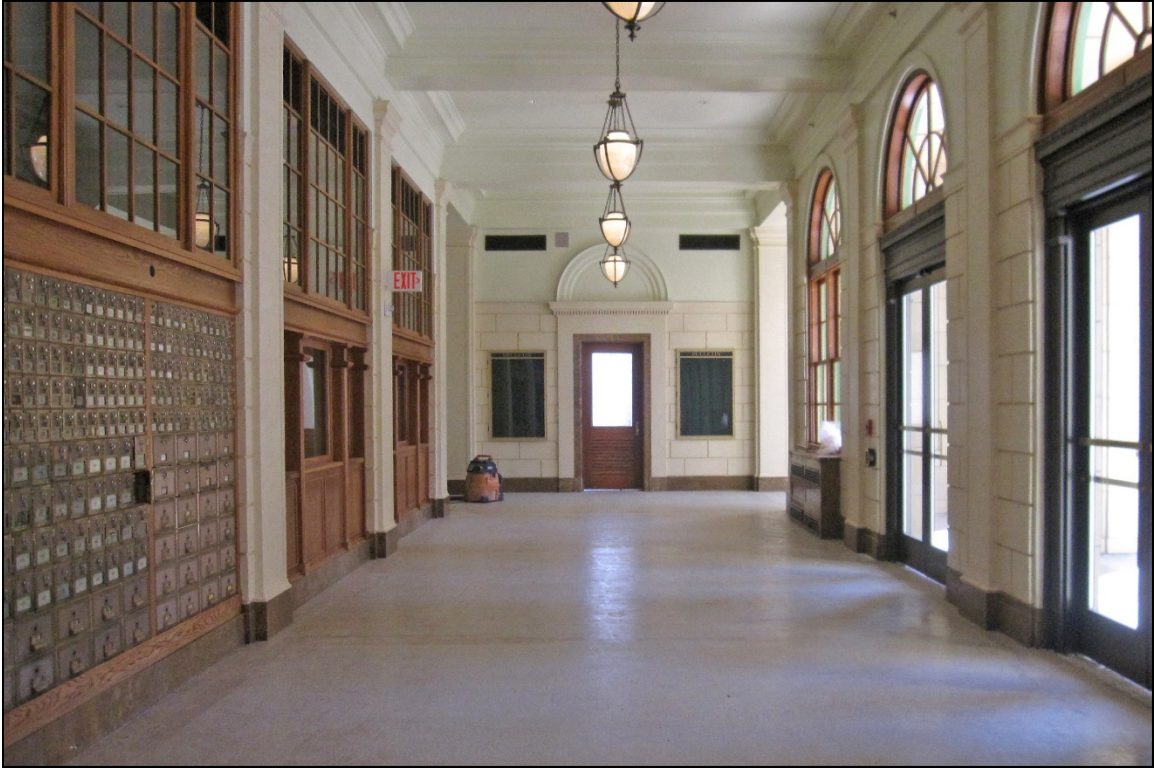
Photograph 27: Lobby, view east
