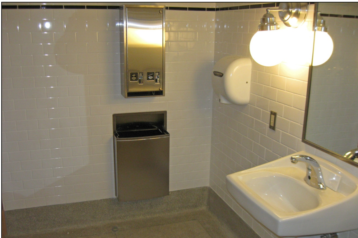
Photograph 50: Family restroom, view southwest
