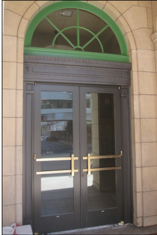
Photograph 11: New entrance doors at Loggia, view north
