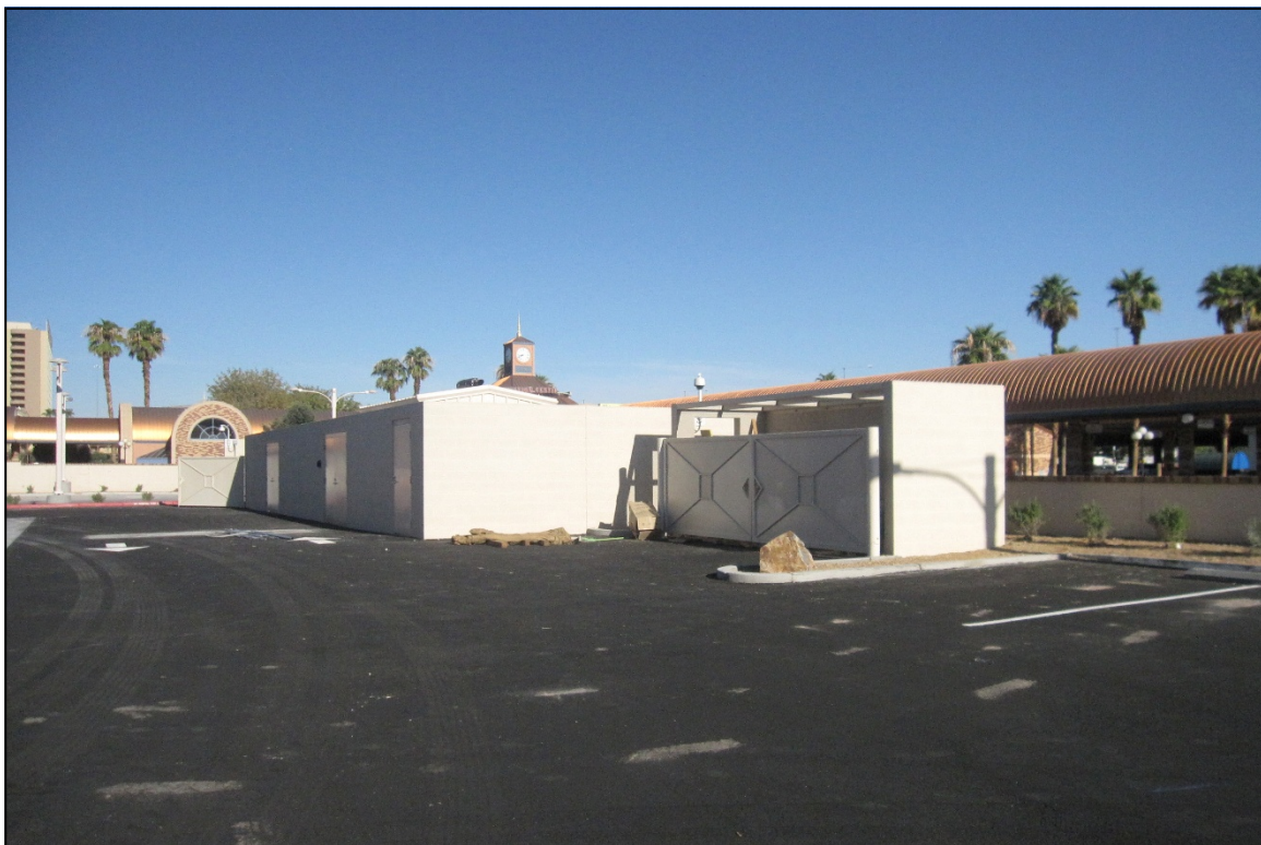
Photograph 7: Mechanical and trash enclosures, view northwest
