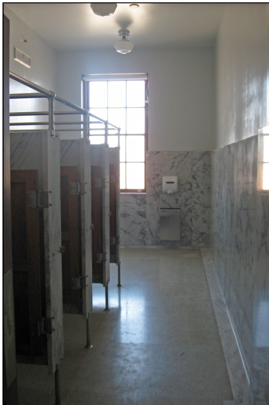
Photograph 72: Women's restroom, view north
