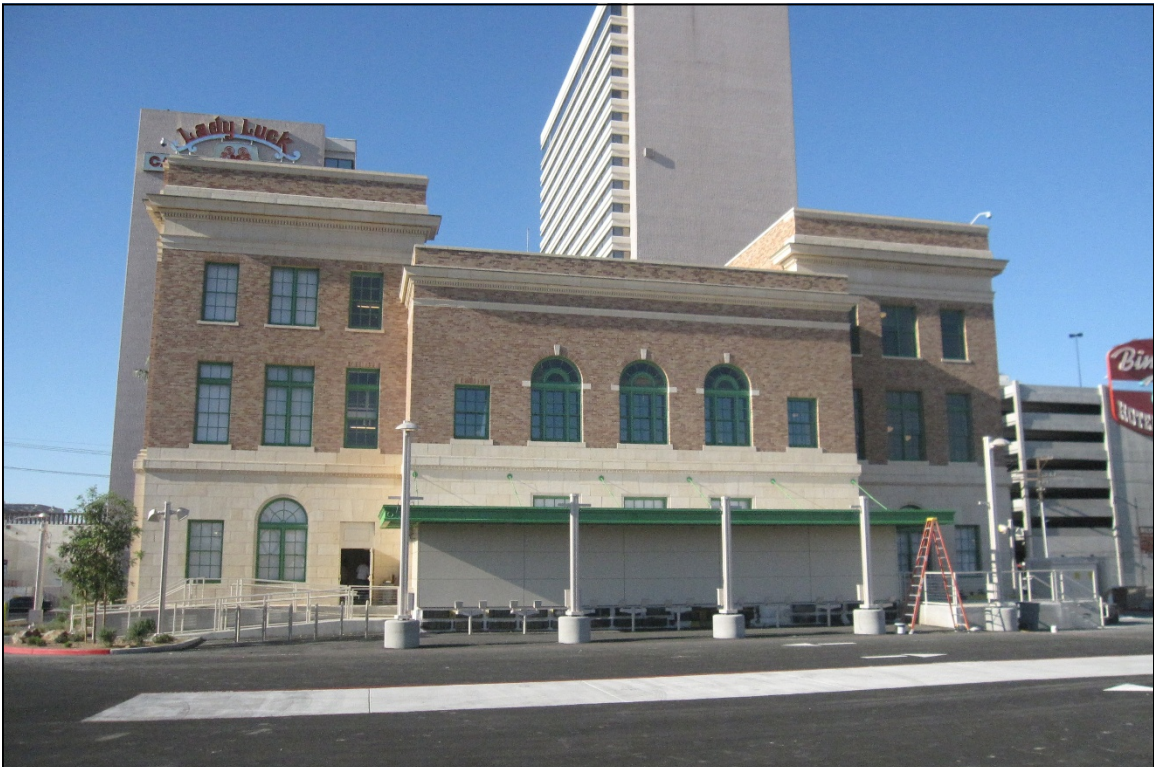
Photograph 4: North elevation, view south
