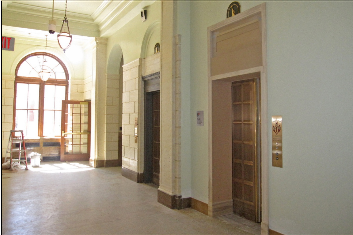
Photograph 23: Lobby, view southwest, note new elevator at right
