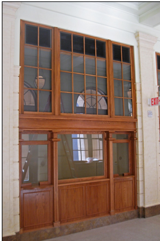
Photograph 30: Detail of new ticket booth, view north
