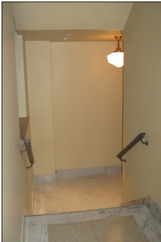
Photograph 14: Stair 1 to basement, view west
