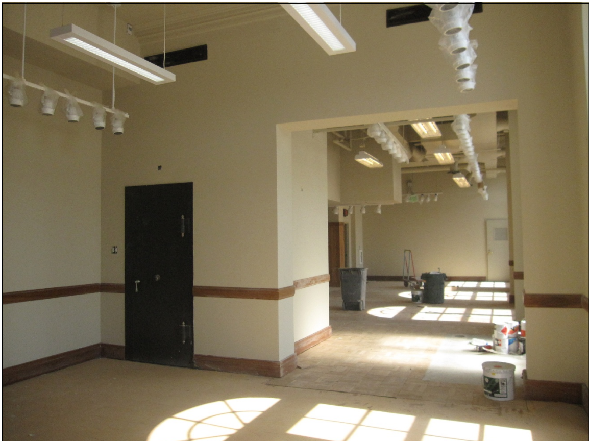
Photograph 34: Retail area, view northwest
