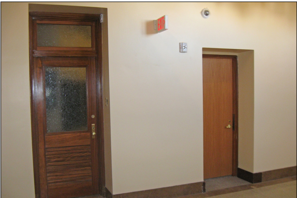
Photograph 60: Third floor corridor, view south
