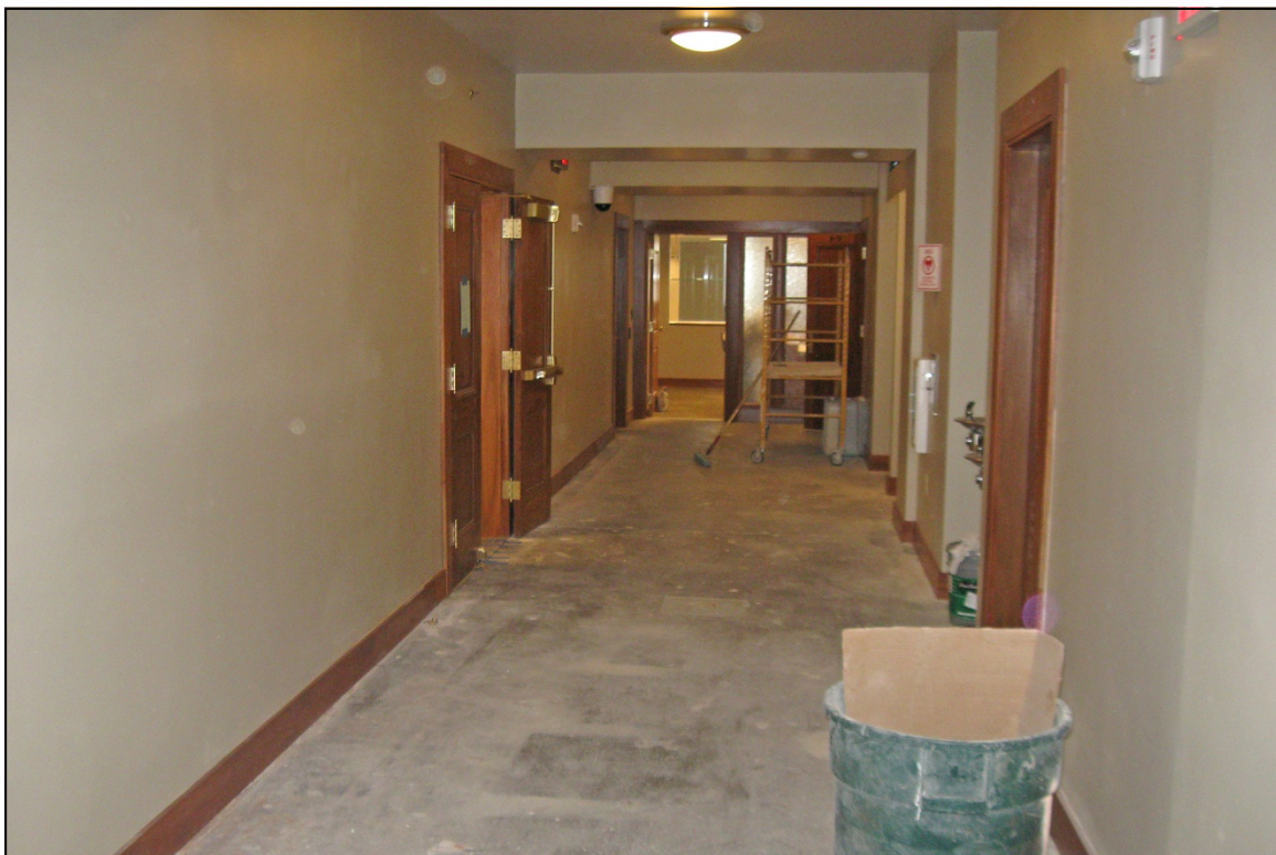
Photograph 17: Basement corridor, view east
