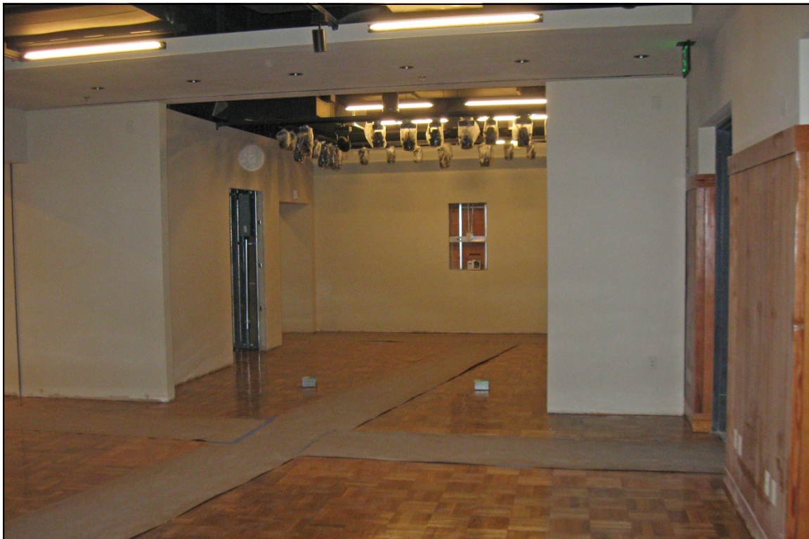
Photograph 40: Exhibit area, view west
