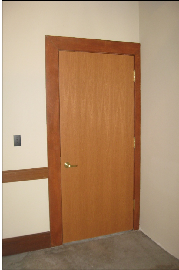
Photograph 67: New door in exhibit area, view north
