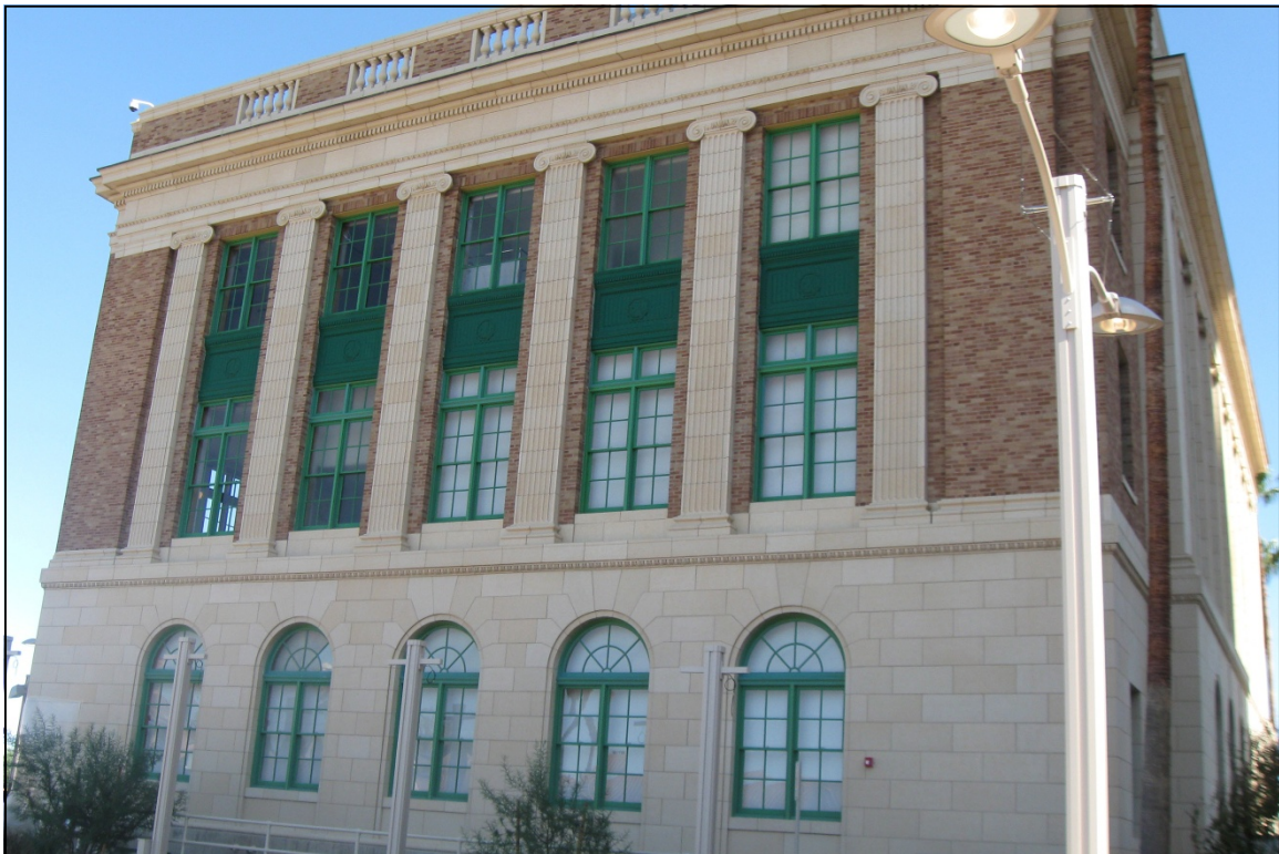
Photograph 2: East elevation, view east
