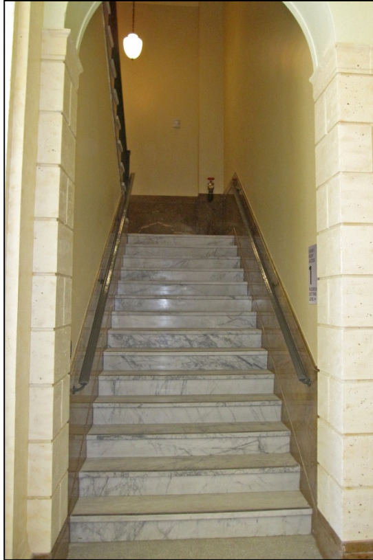
Photograph 25: Stair 1 from lobby to second floor, view west
