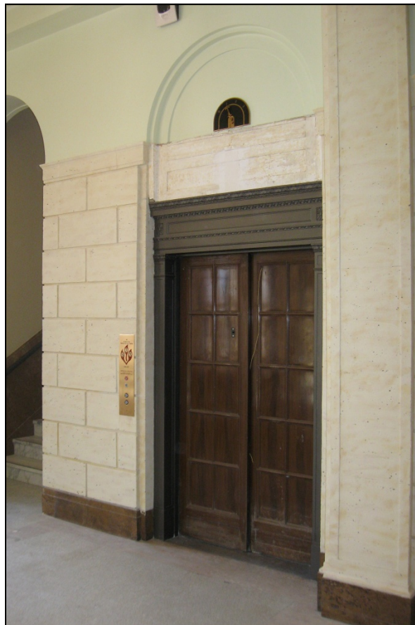
Photograph 24: Historic elevator at lobby, view southwest
