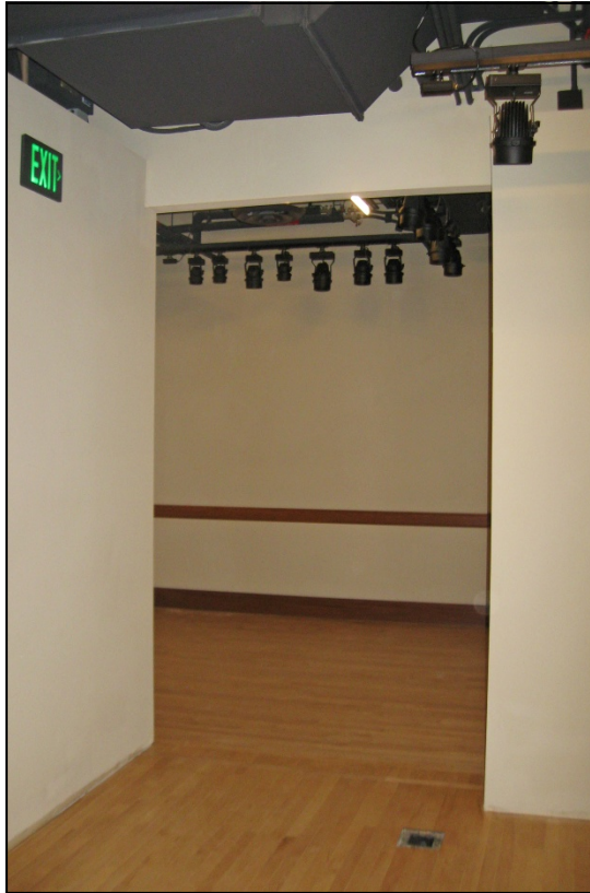
Photograph 53: Enlarged doorway in exhibit area, view east
