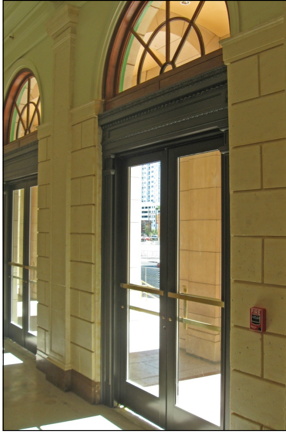
Photograph 21: Lobby entrance doors , view southeast
