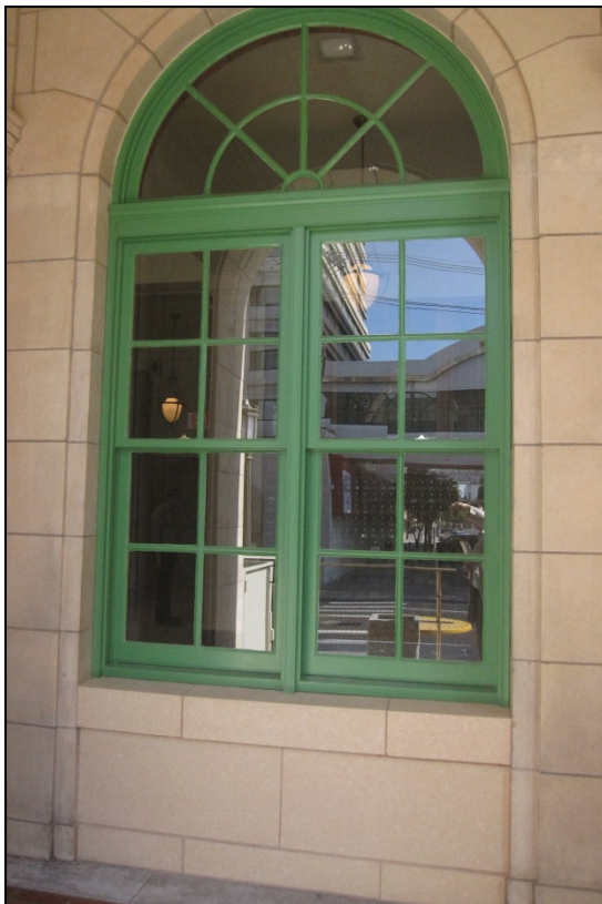
Photograph 12: New window and terra cotta bulk-head at Loggia, previously a door, view north
