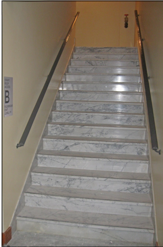
Photograph 15: Stair 1 at basement, view west
