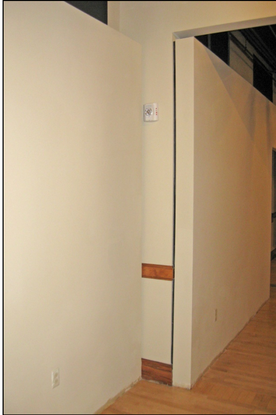
Photograph 55: Exhibit wall at header/wing wall opening, view southwest, note typical detail
