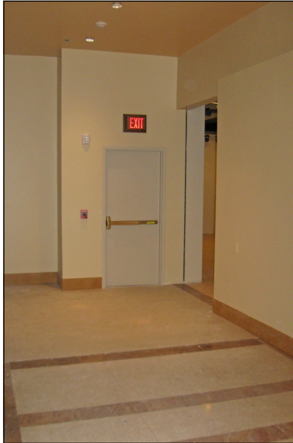
Photograph 45: Second floor corridor, view north, note door to Stair 2
