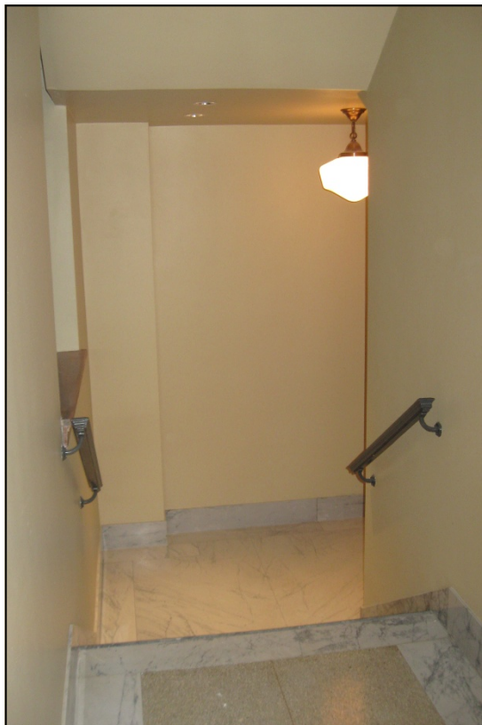
Photograph 14: Stair 1 to basement, view west
