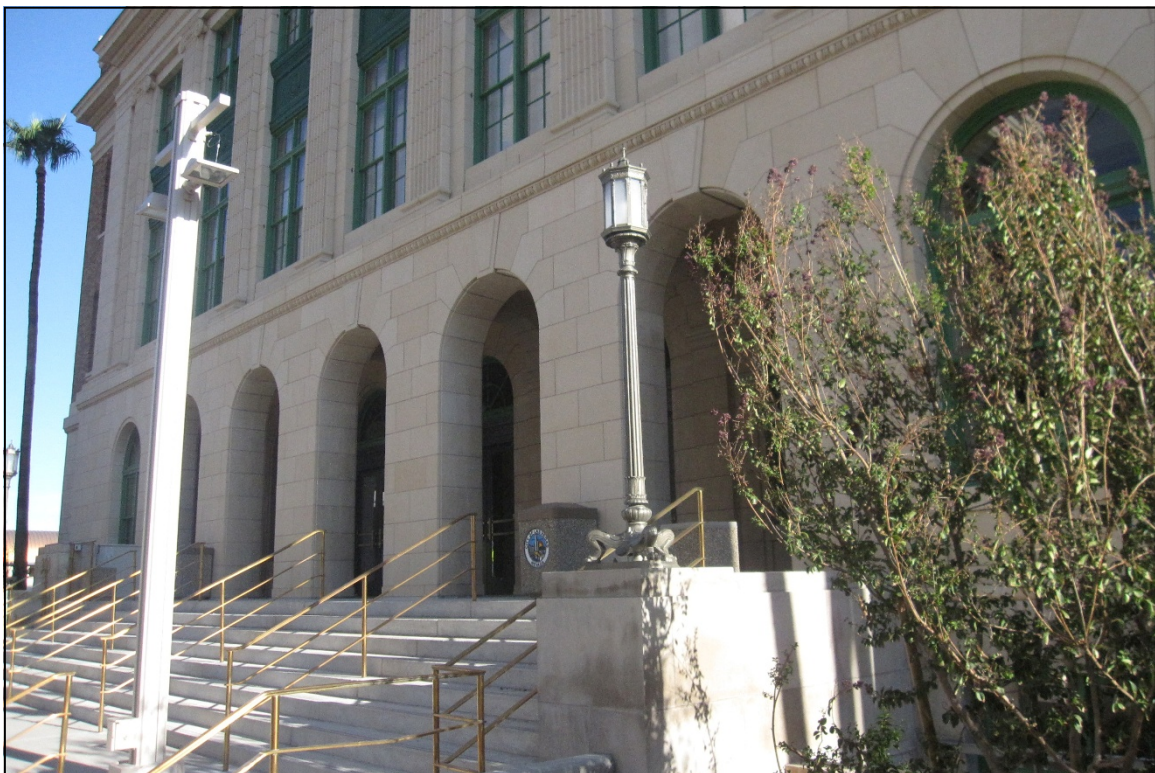
Photograph 8: Loggia, south façade, view northwest
