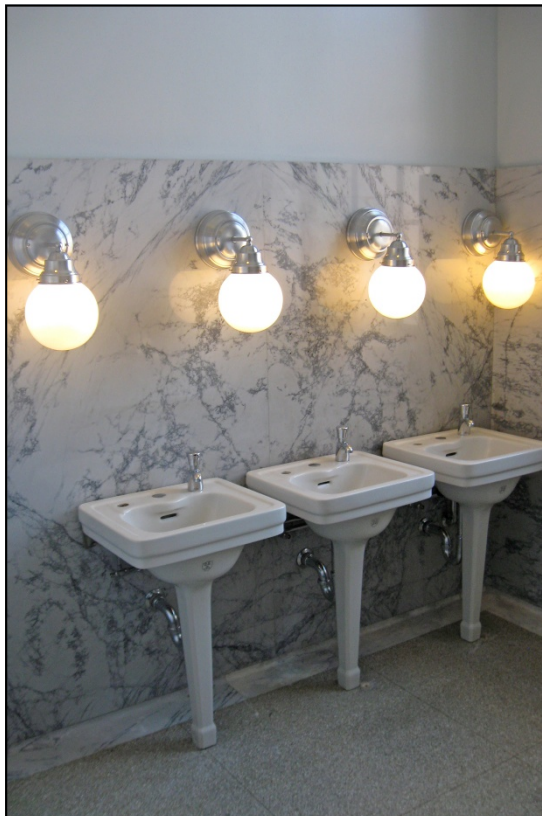
Photograph 74: Women's restroom sinks, view northwest
