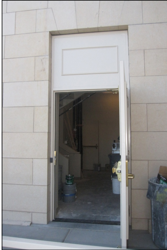
Photograph 13: New exit door at Stair 2, previously a window, north elevation, view south
