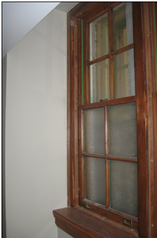
Photograph 16: Window at basement, view south-east
