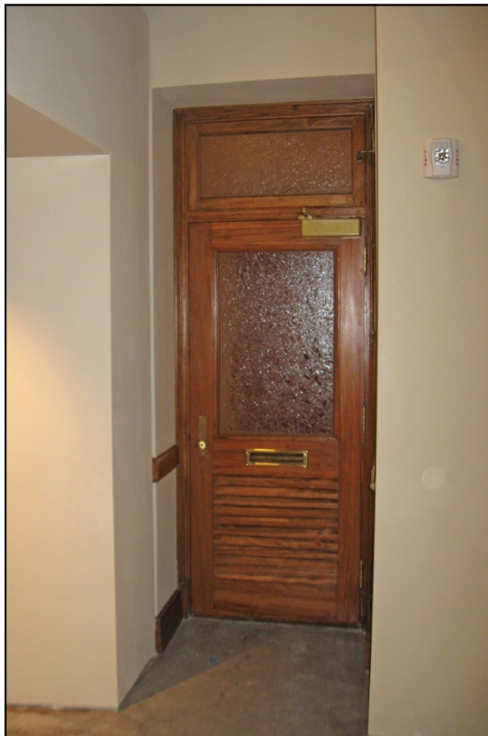
Photograph 56: Historic door in exhibit area, view north,
