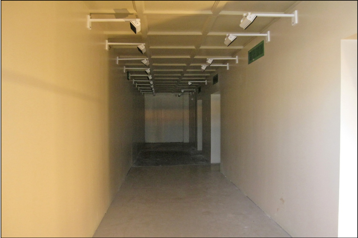
Photograph 41: Enclosed loading dock, view east
