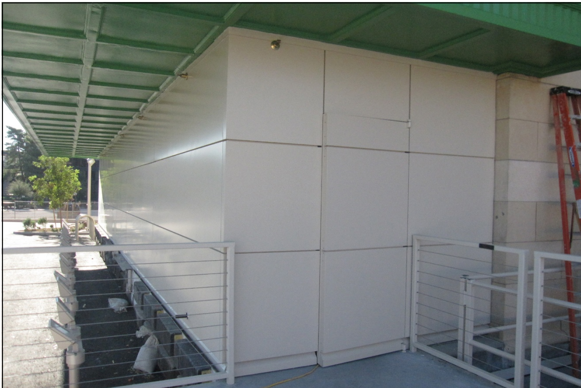
Photograph 6: Loading dock enclosure door, view southeast
