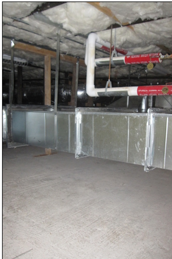
Photograph 80: Attic with new ductwork and insulation, view east
