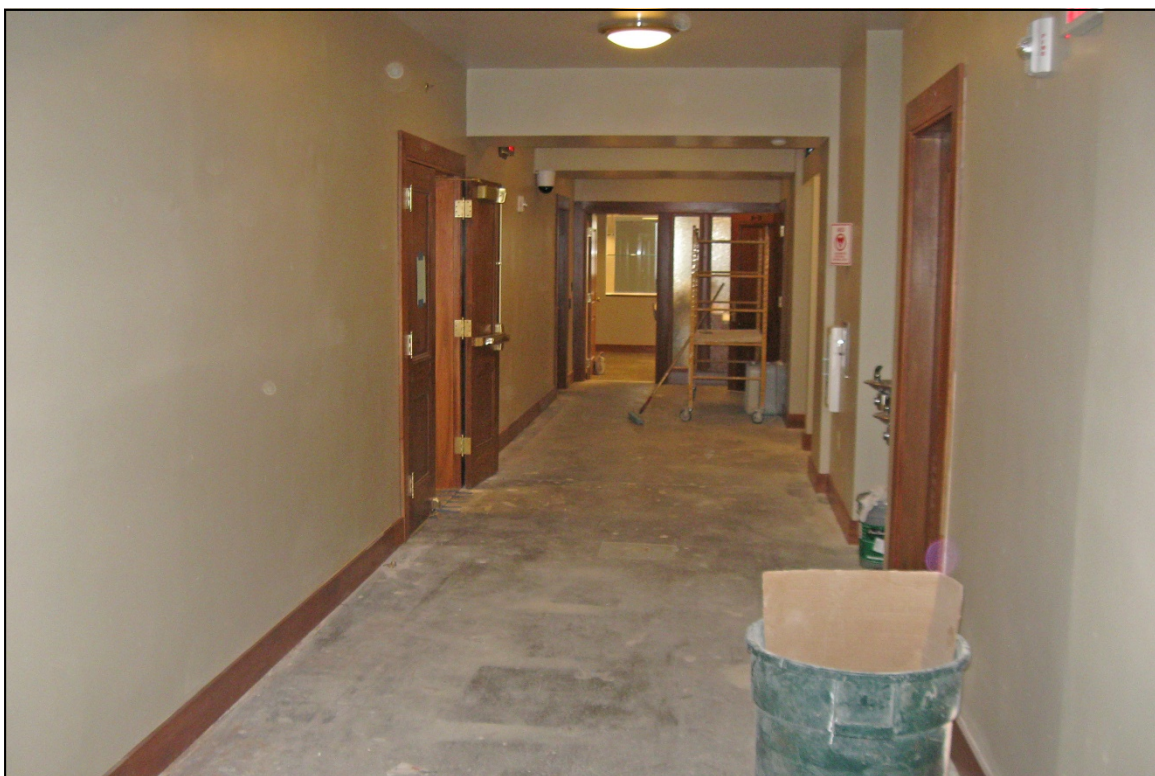
Photograph 17: Basement corridor, view east
