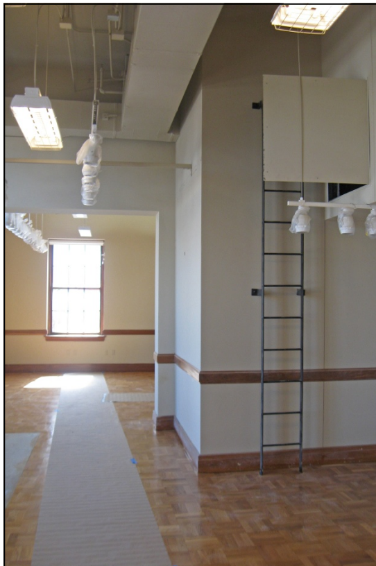
Photograph 36: Retail area, view south, note re-installed ladder to "eye in the sky"
