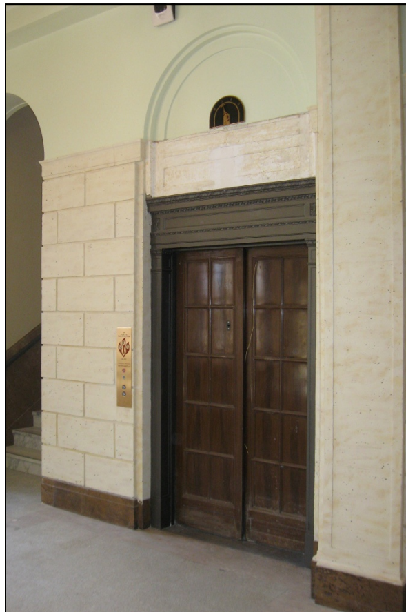
Photograph 24: Historic elevator at lobby, view southwest
