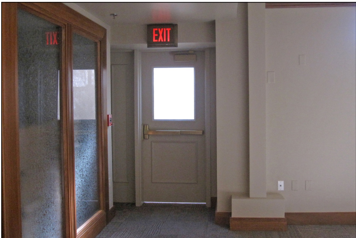
Photograph 18: New exit door in museum office at basement, previously a window, view east
