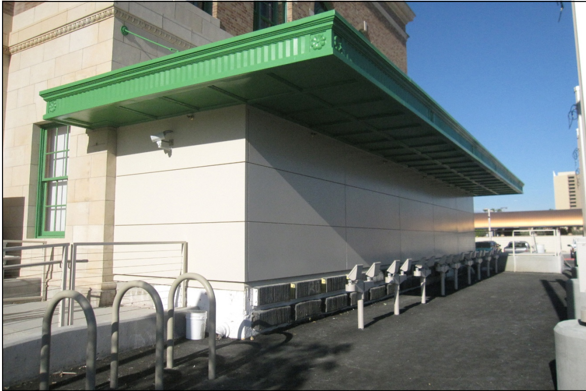
Photograph 5: Loading dock enclosure, southwest
