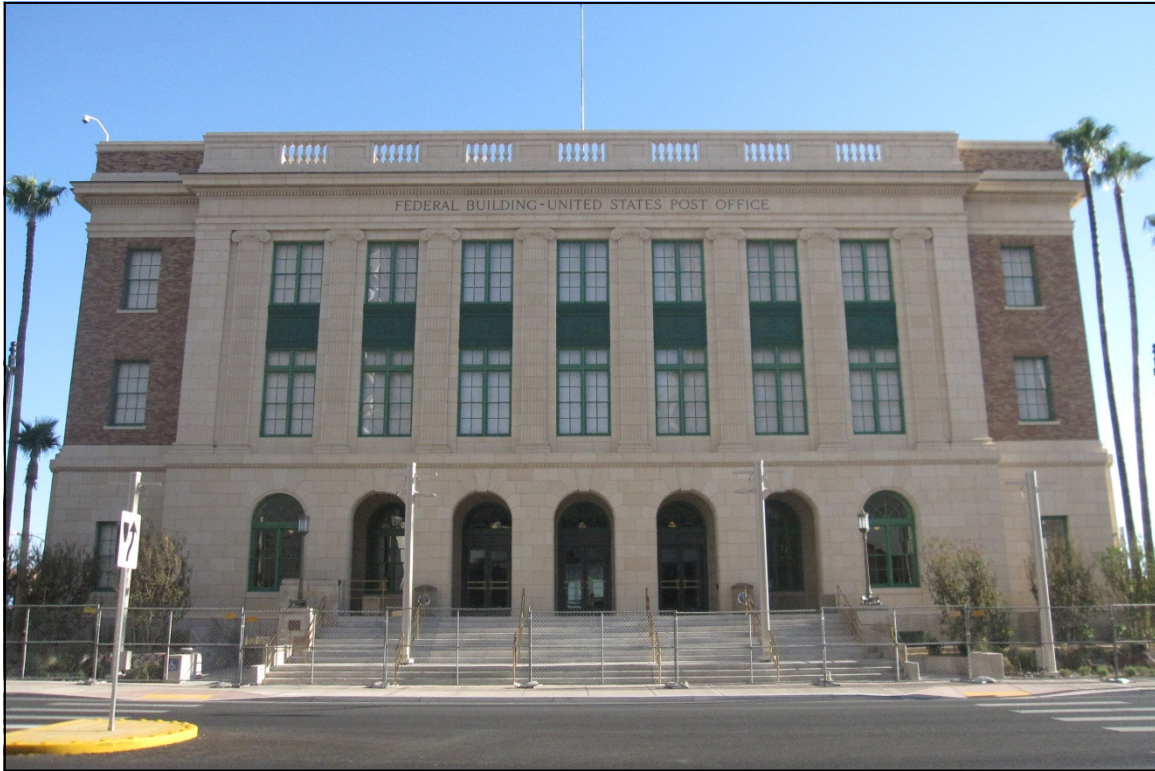
Photograph 1: South façade, view north
