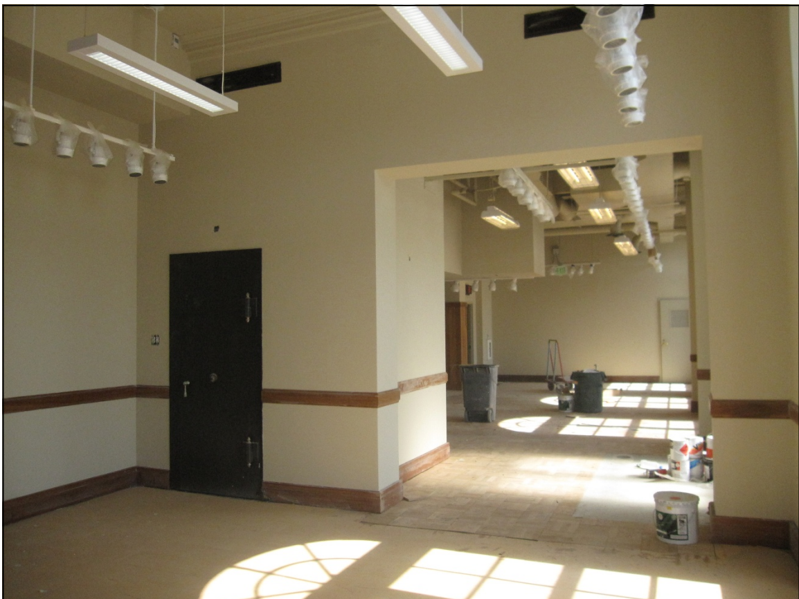
Photograph 34: Retail area, view northwest
