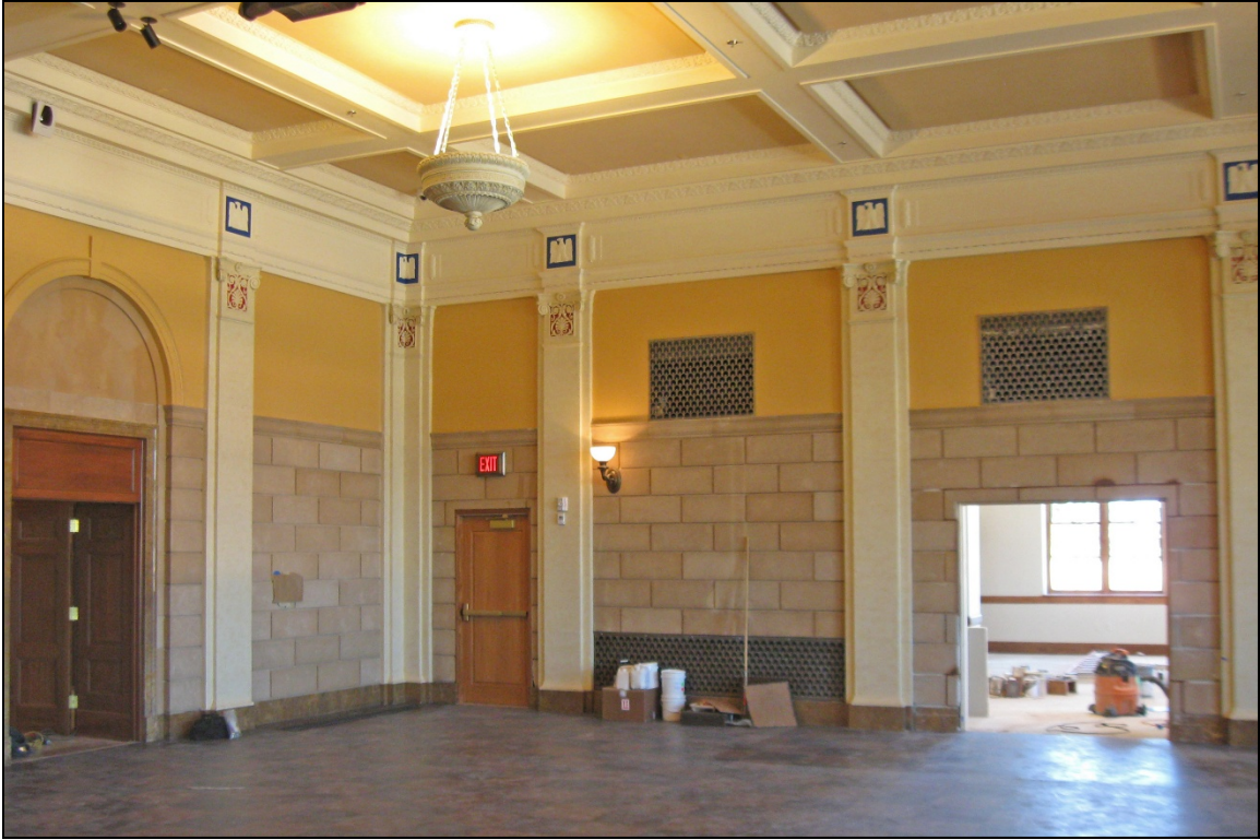
Photograph 47: Courtroom, southwest, note widened exit door on left and new double door opening on right
