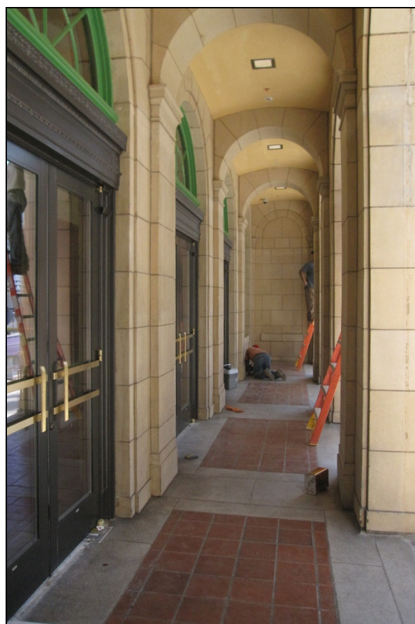
Photograph 10: Loggia, south façade, view east
