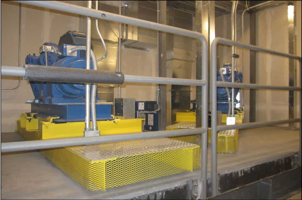
Photograph 81: Elevator machine room, view northwest
