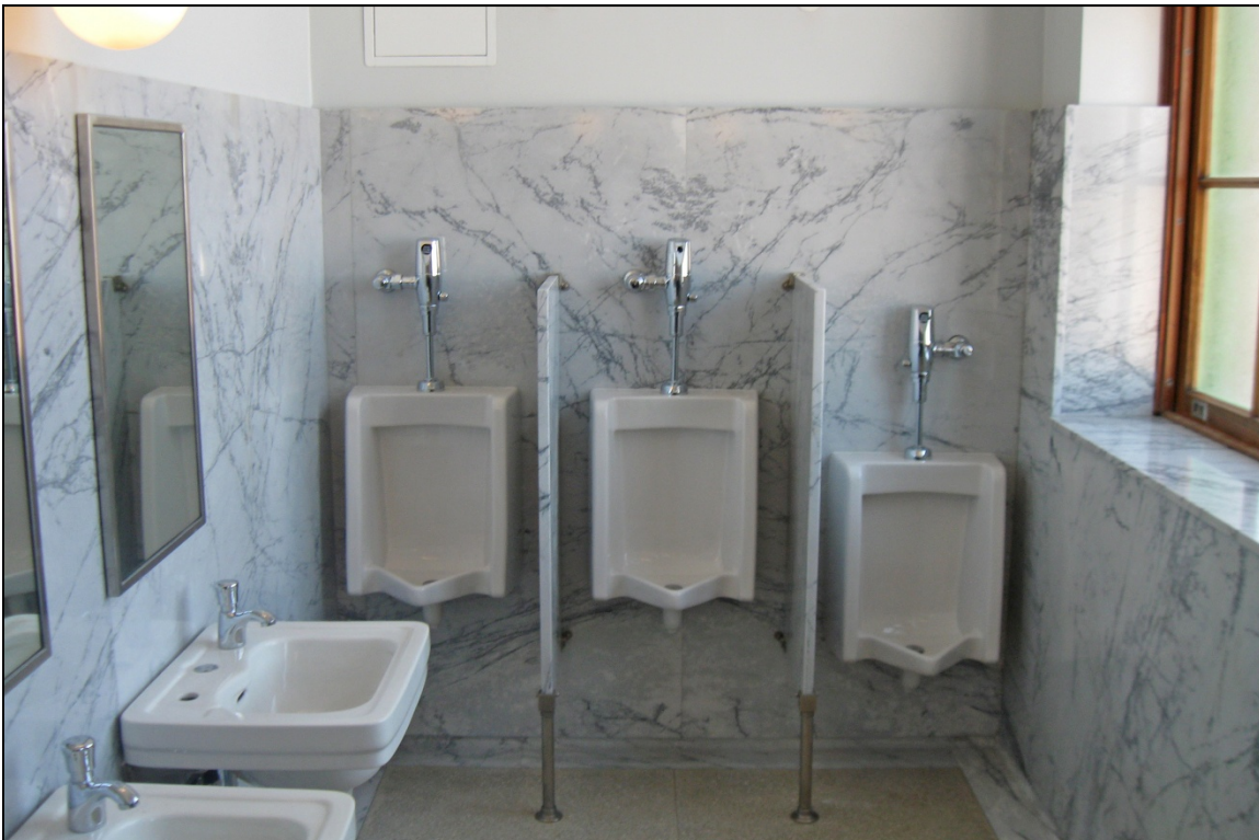
Photograph 78: Men's restroom, view south
