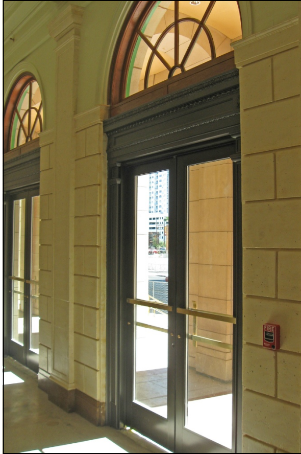
Photograph 21: Lobby entrance doors , view southeast
