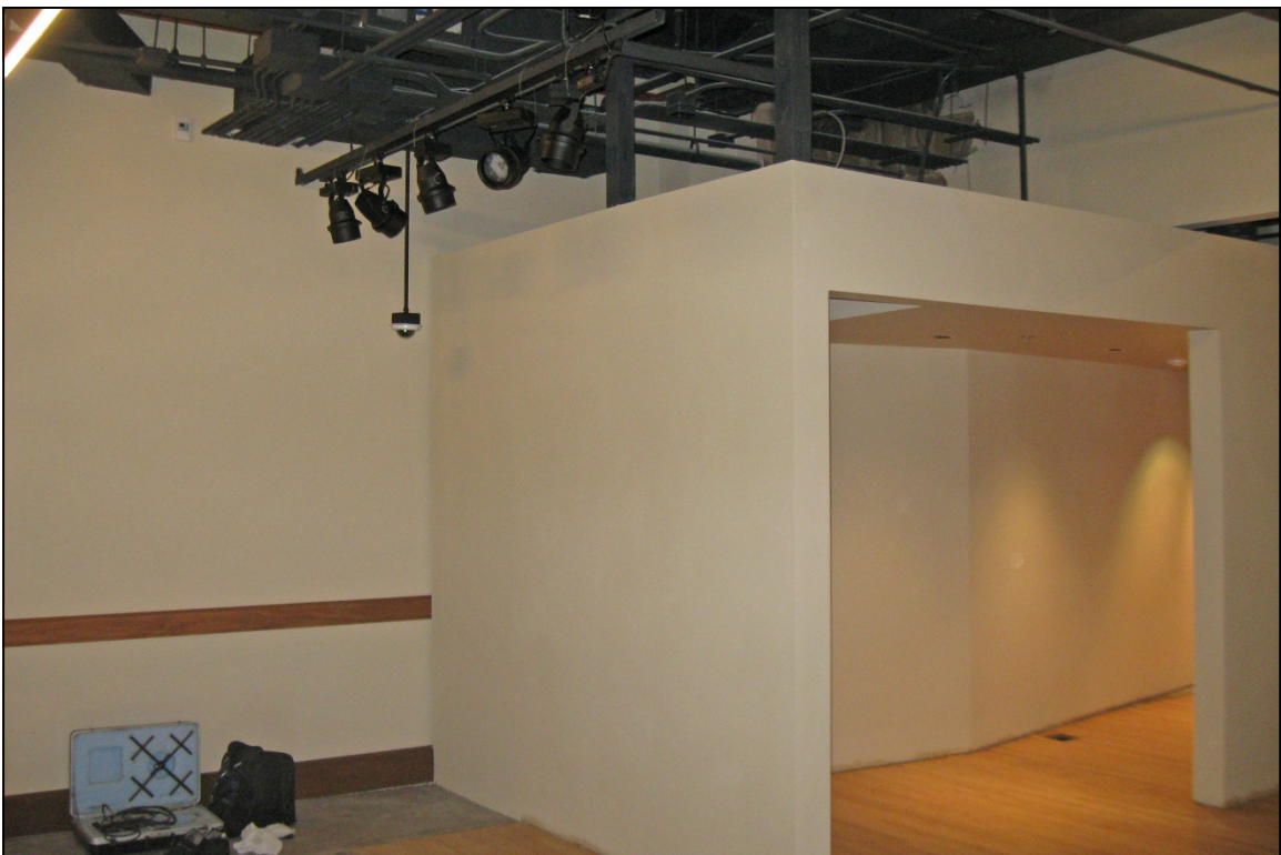
Photograph 58: Exhibit area, view northeast
