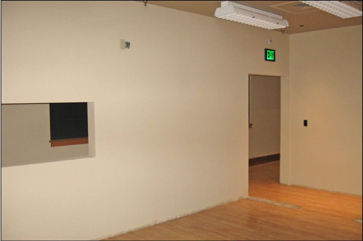
Photograph 65: Exhibit area, view southwest
