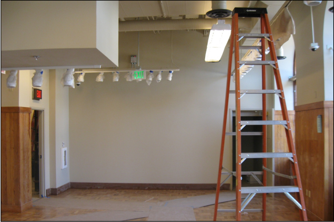
Photograph 37: Retail area, view north
