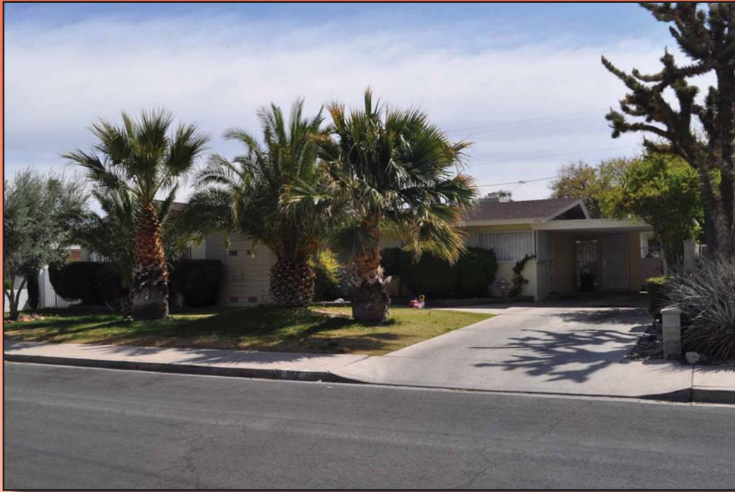
Figure 4.43 552 Canosa Avenue designed by William Leavers, architect.
