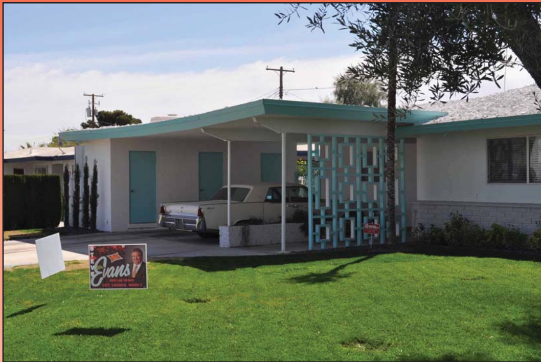
Figure 4.37 548 Barbara Way by Jack Belcher, architect (with Tropicool Roof).
