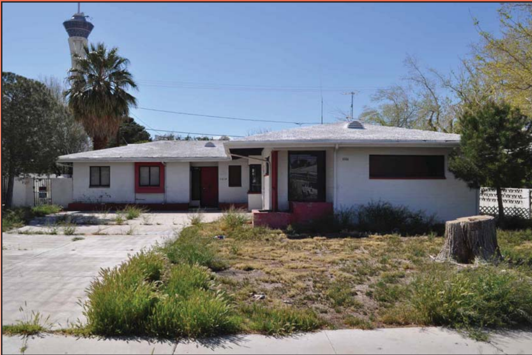
Figure 3.46 Example of a converted garage at 1814 S. 6th Street.
