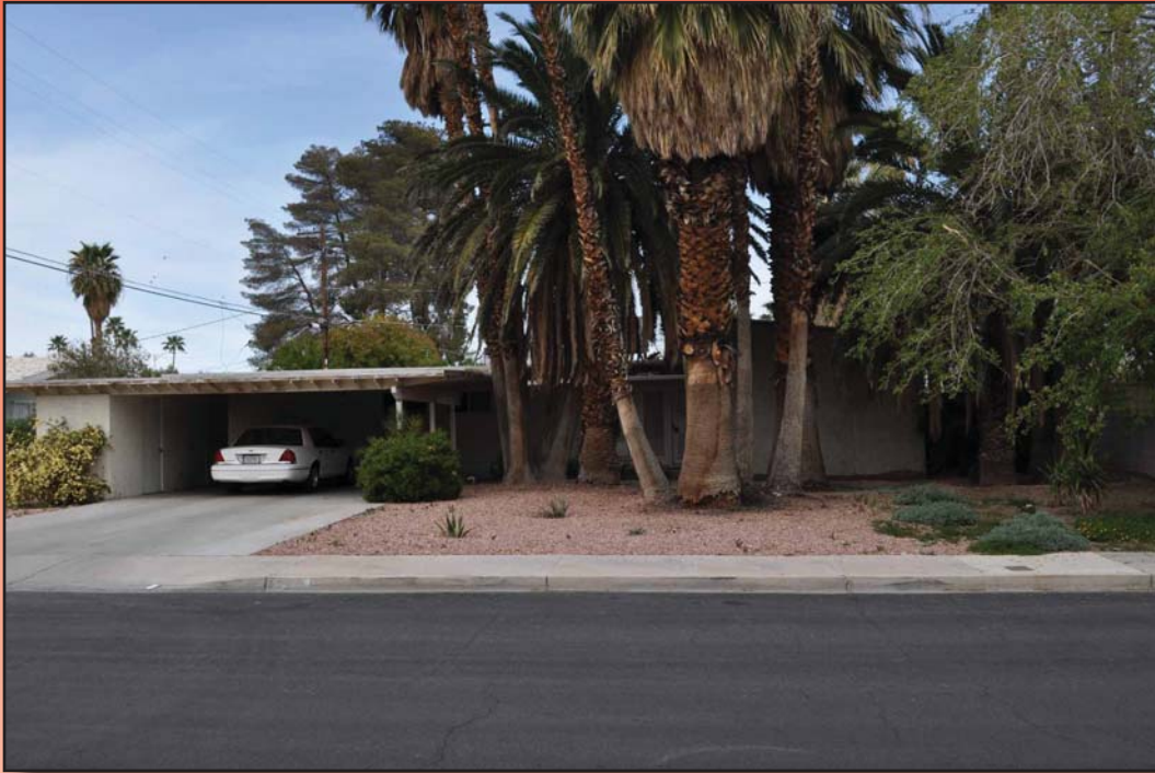
Figure 4.5 Post-World War II Contemporary style with International style influences at 547 Canosa Avenue (Jack Knighton, architect).
