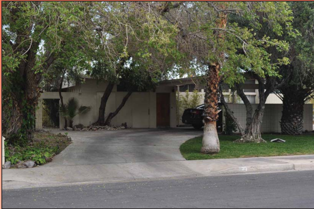
Figure 4.45 549 Canosa Avenue designed by Hugh Taylor, architect.
