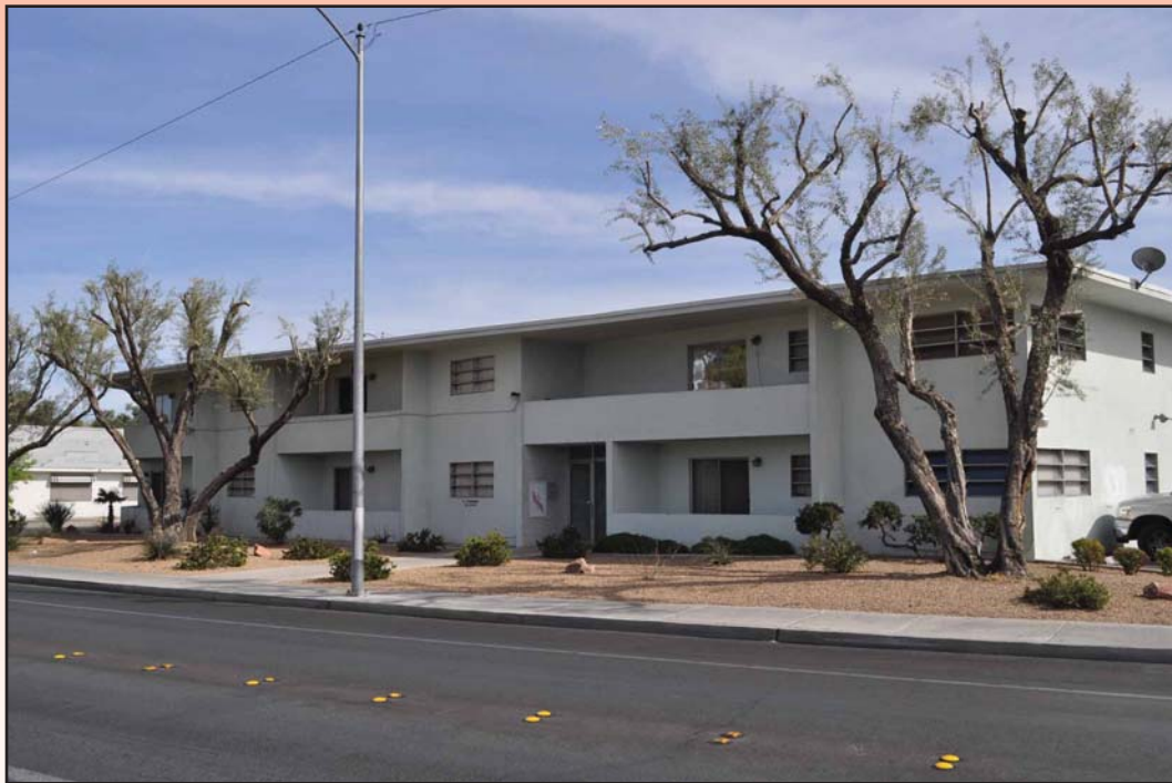
Figure 4.8 International-style Rexford Apartments at 1700 Rexford Drive (Jack Knighton, architect).
