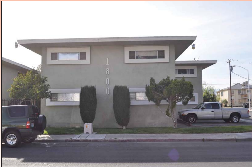
Figure 4.50 Eight-unit apartment recommended eligible at 1800 Rexford Drive.
