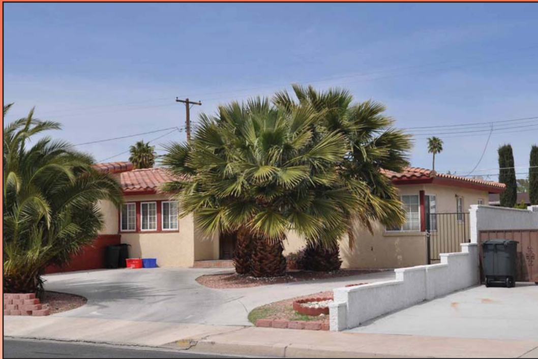
Figure 4.33 New windows, garage, and tile roof at 544 Canosa Way.
