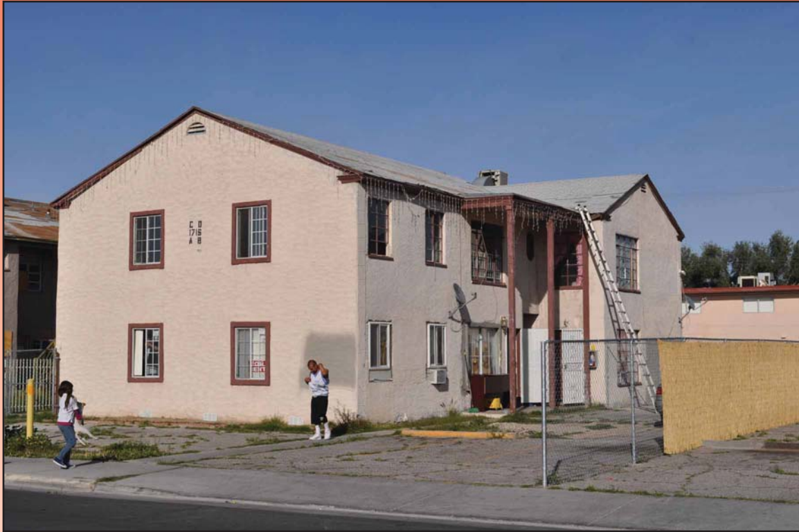
Figure 4.53 Four-plex recommended not eligible at 1717 Santa Paula Drive.
