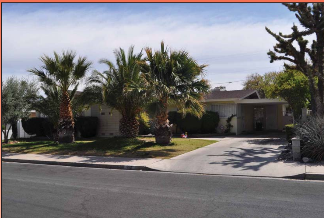
Figure 4.43 552 Canosa Avenue designed by William Leavers, architect.
