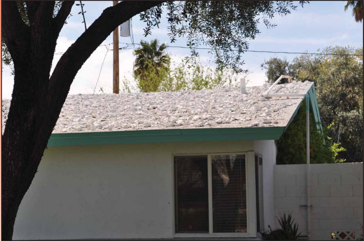
Figure 4.11 Close up of a Tropicool roof at 548 Barbara Way.
