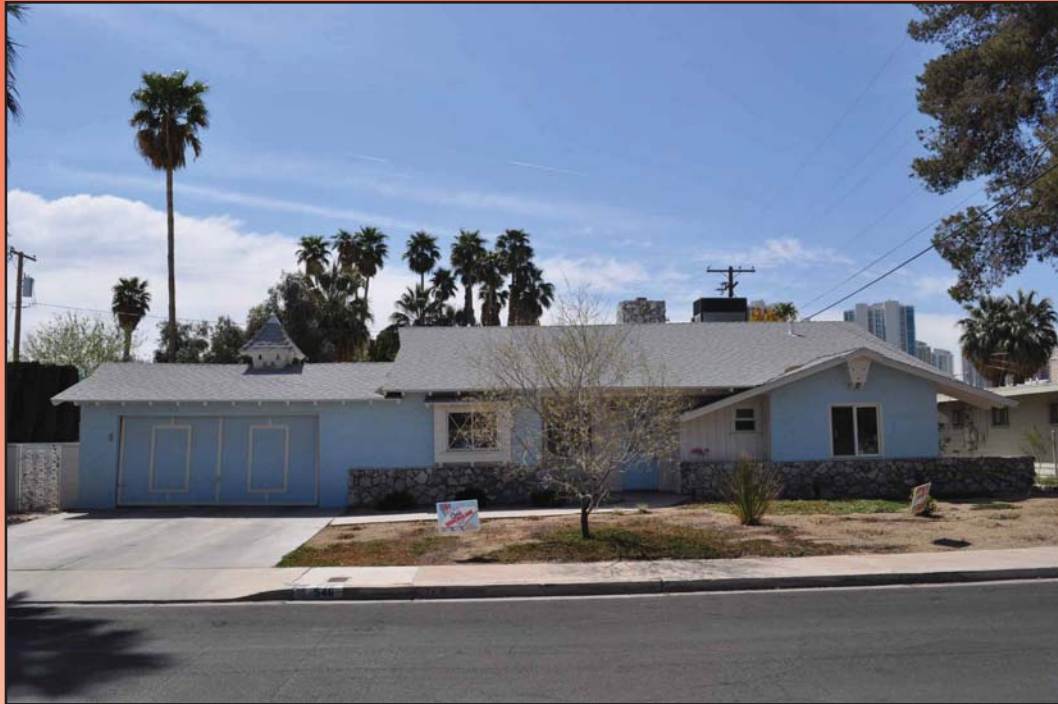
Figure 4.7 Character ranch at 546 Barbara Way (Hugh Taylor, architect).
