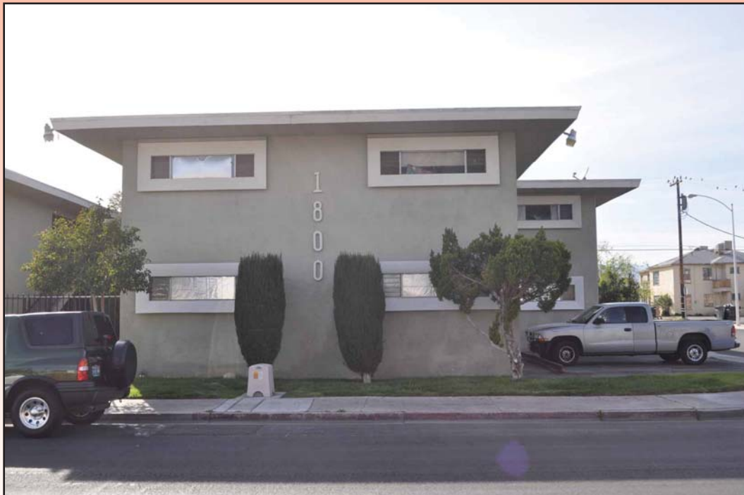
Figure 4.50 Eight-unit apartment recommended eligible at 1800 Rexford Drive.
