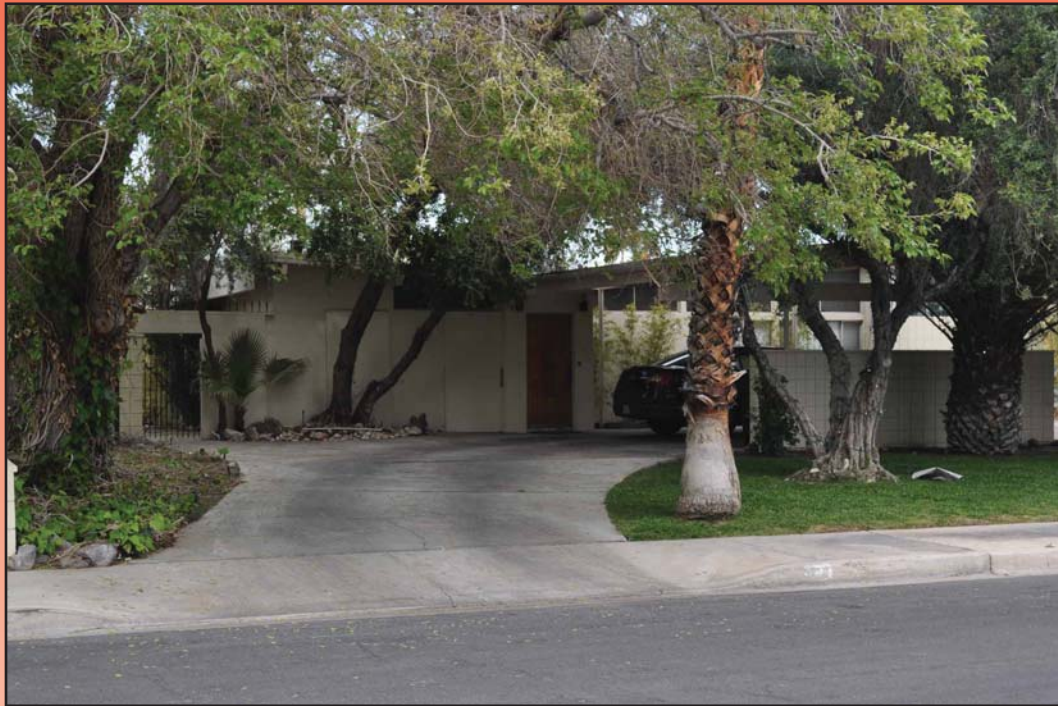
Figure 4.45 549 Canosa Avenue designed by Hugh Taylor, architect.
