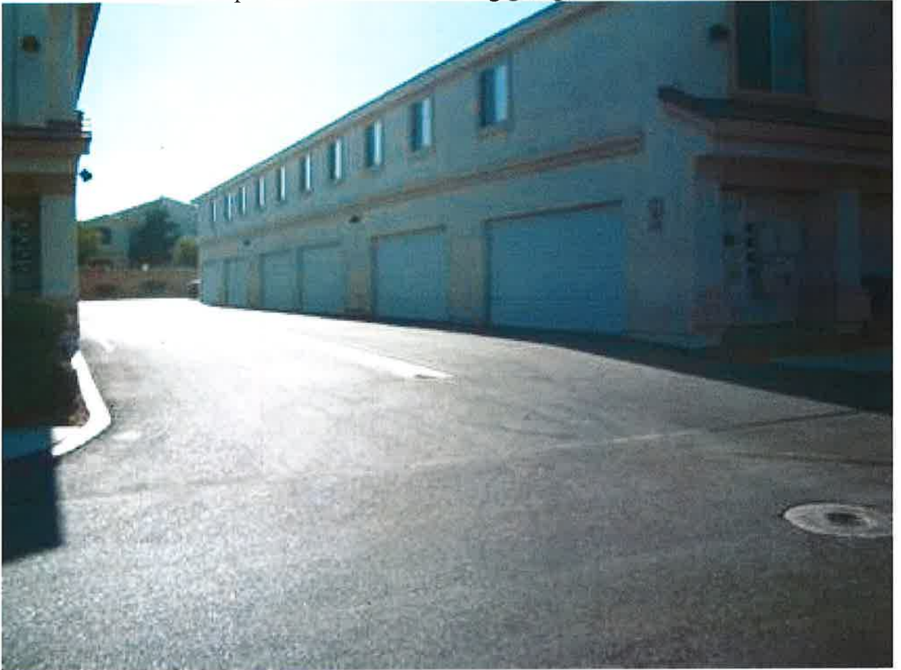
Rear of Apartment Homes showing garage entrance
