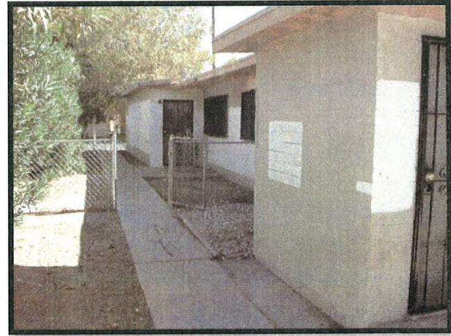
North view sidewalk to unit C
