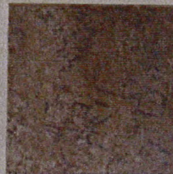
Toilet Room Wall Tile
