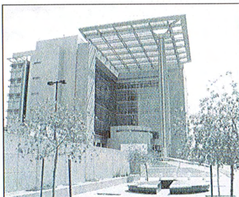
PHOTO 6: FEDERAL BUILDING / U.S. COURTHOUSE
