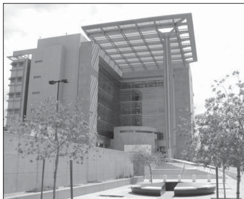
PHOTO 6: FEDERAL BUILDING / U.S. COURTHOUSE
