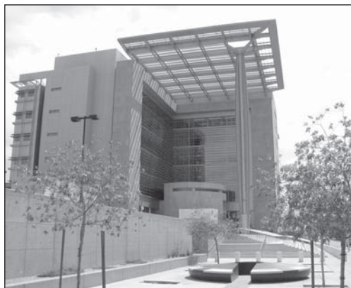
PHOTO 6: FEDERAL BUILDING / U.S. COURTHOUSE
