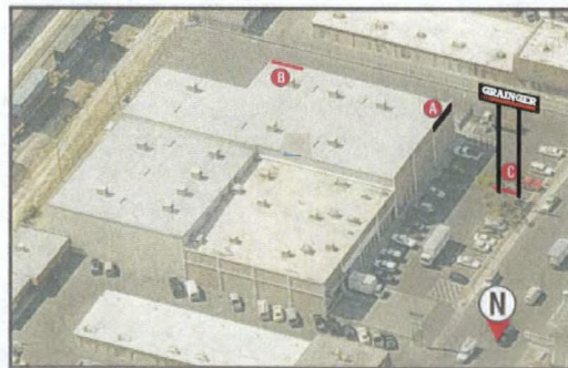
Aerial View- Site Location Showing Signs
