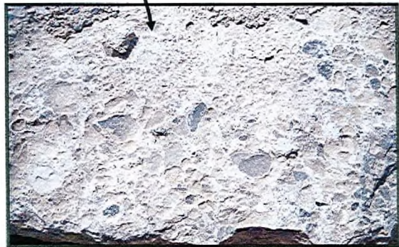
STONE FACADE NATURAL CALICHE ROCK COLLECTED ON-SITE & SET IN MORTAR
