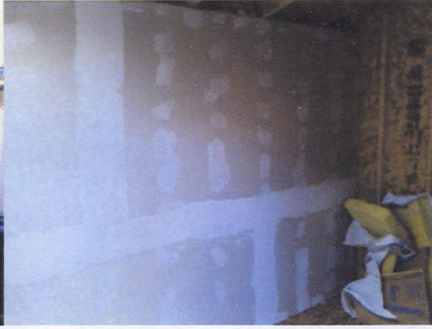
Firewall on side facing neighbor's wall
