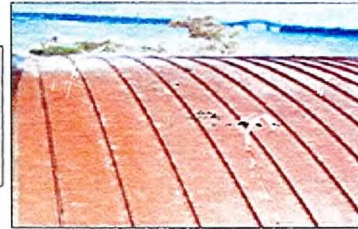
STANDING SEAM COPPER ROOFING
