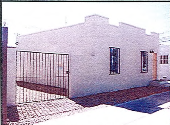
West Southwest Elevation
