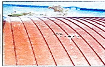
STANDING SEAM COPPER ROOFING
