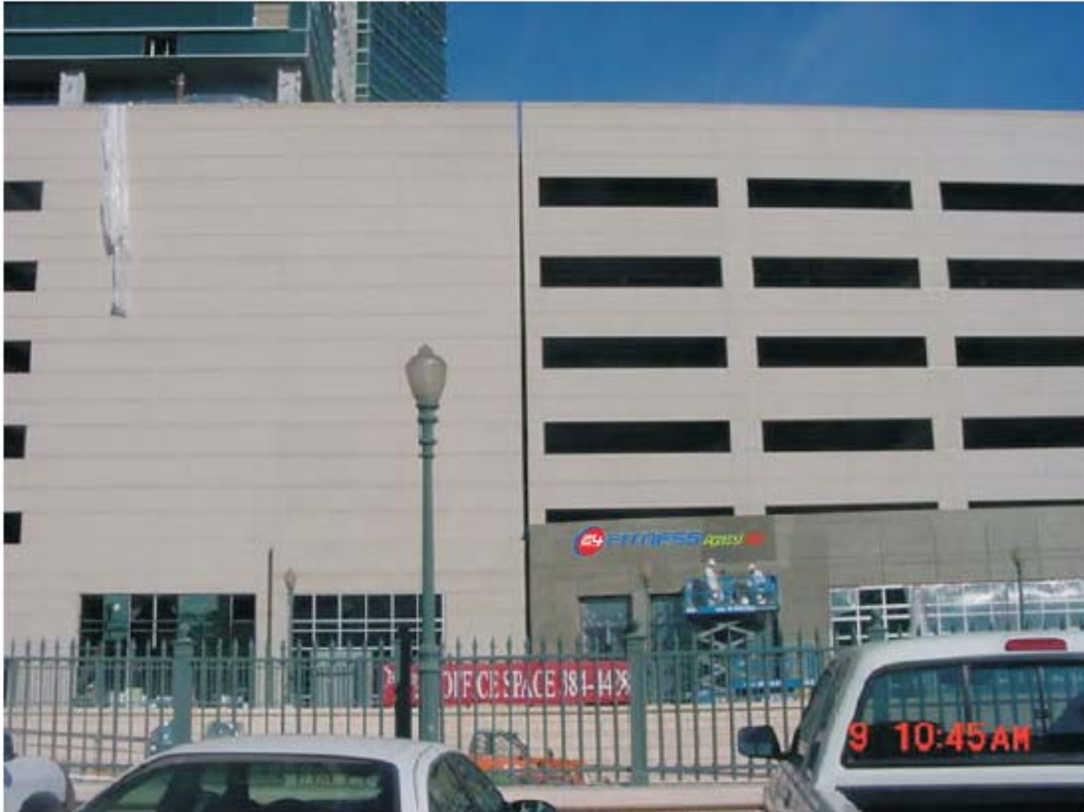
PHOTO OF EXISTING SOUTH ELEVATION
