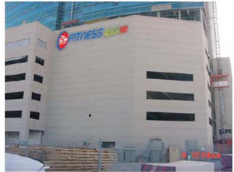
PHOTO OF EXISTING NORTH ELEVATION
