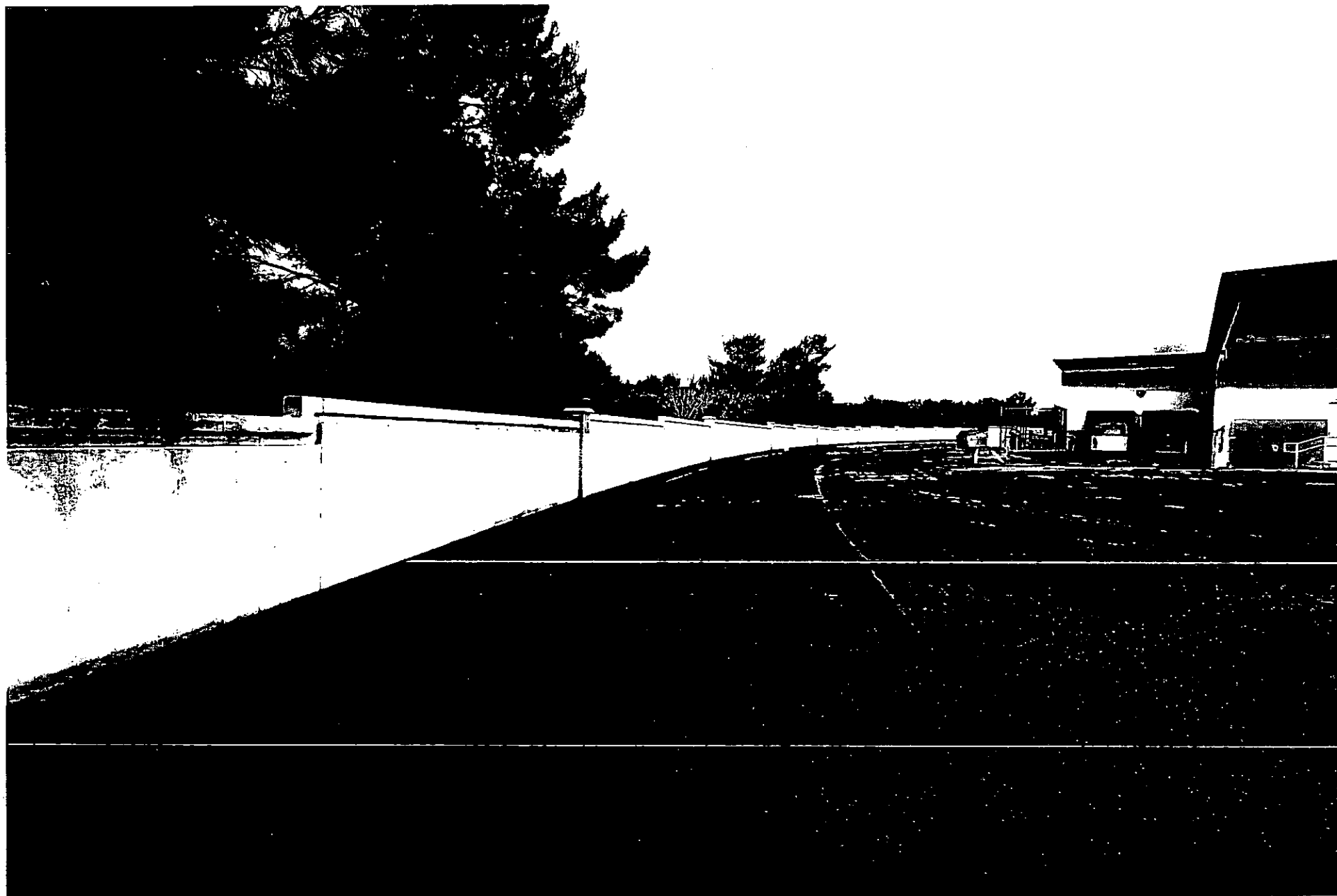
Retain Wall along Drainage Channel TMP-40556
