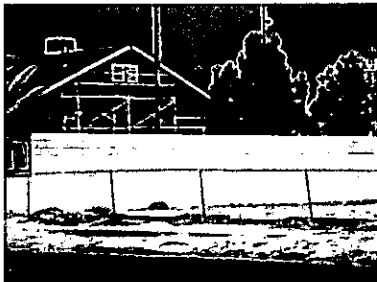
#2 EXISTING FENCE WALL @ NORTH SIDE
