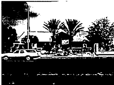
EXISTING LANDSCAPE AT FRONT OF EXISTING BUILDING
