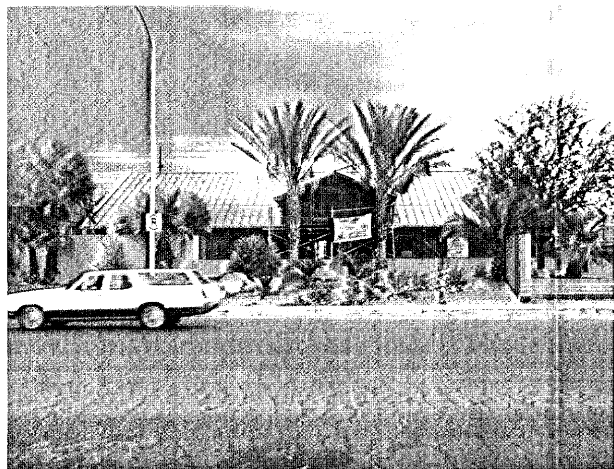
EXISTING LANDSCAPE AT FRONT OF EXISTING BUILDING
