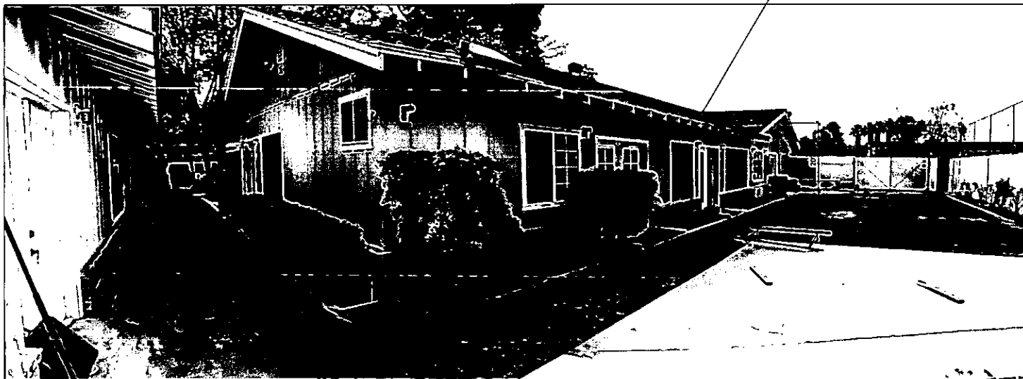
1 NORTH WEST ELEVATION AT 2850 PALOMINO LANE (BUILDING B)
