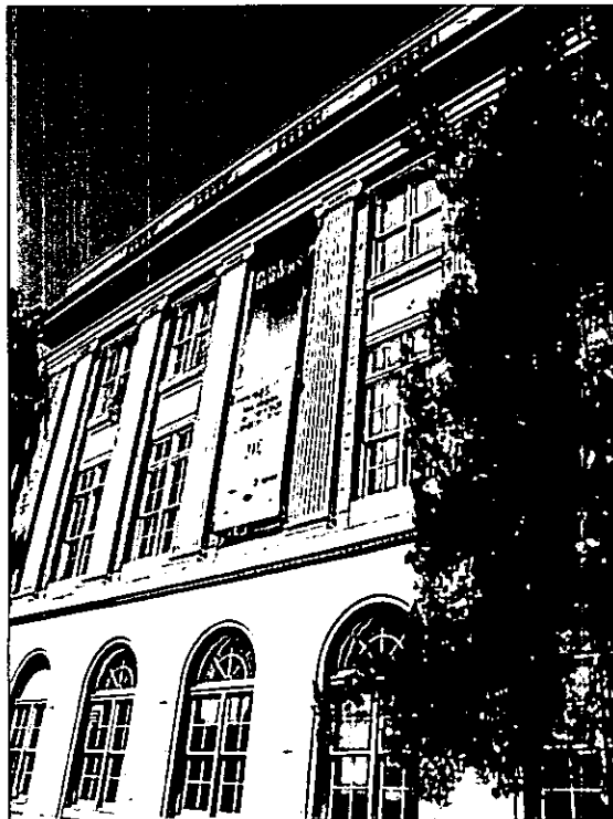
Figure 2: Banner installed on east elevation for Las Vegas Centennial Celebration (2005).
