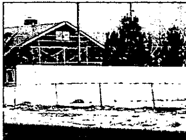
#2 EXISTING FENCE WALL @ NORTH SIDE
