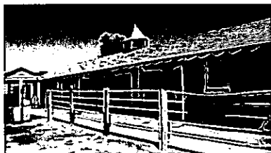
Bldg. 6: stables (milk barn)
