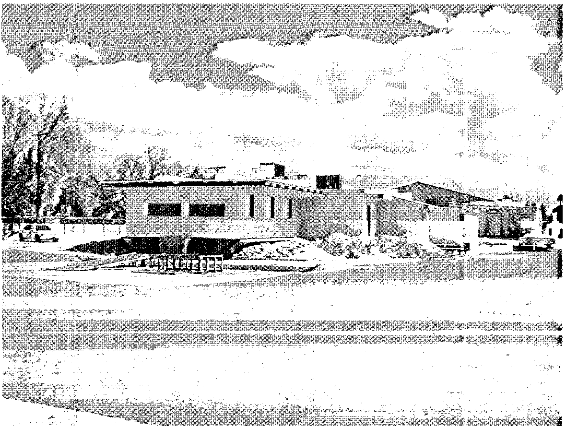
BUILDING "A" AND "B" FROM THE NORTH
