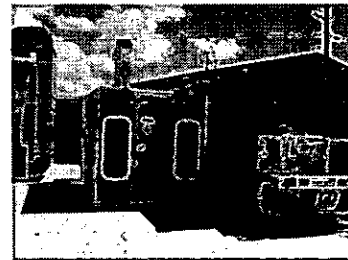
BUILDING "D" MIXING BOOTH
