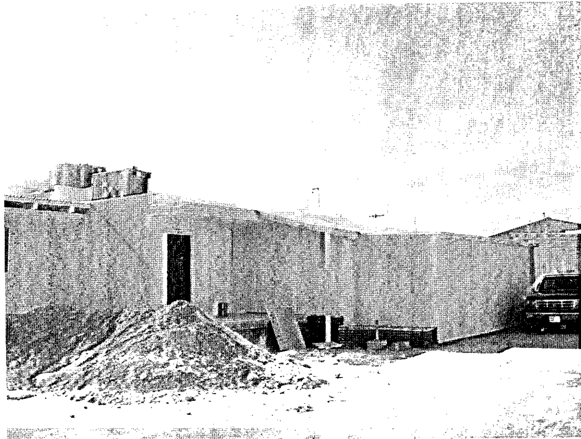
BUILDING "A" WEST SIDE
