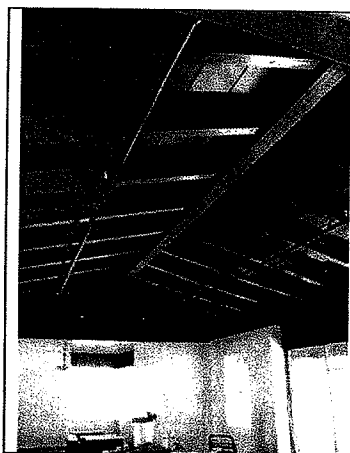
1. The visually intrusive pipes on the ceiling of the Foreman's House were removed during renovation. [crop]
