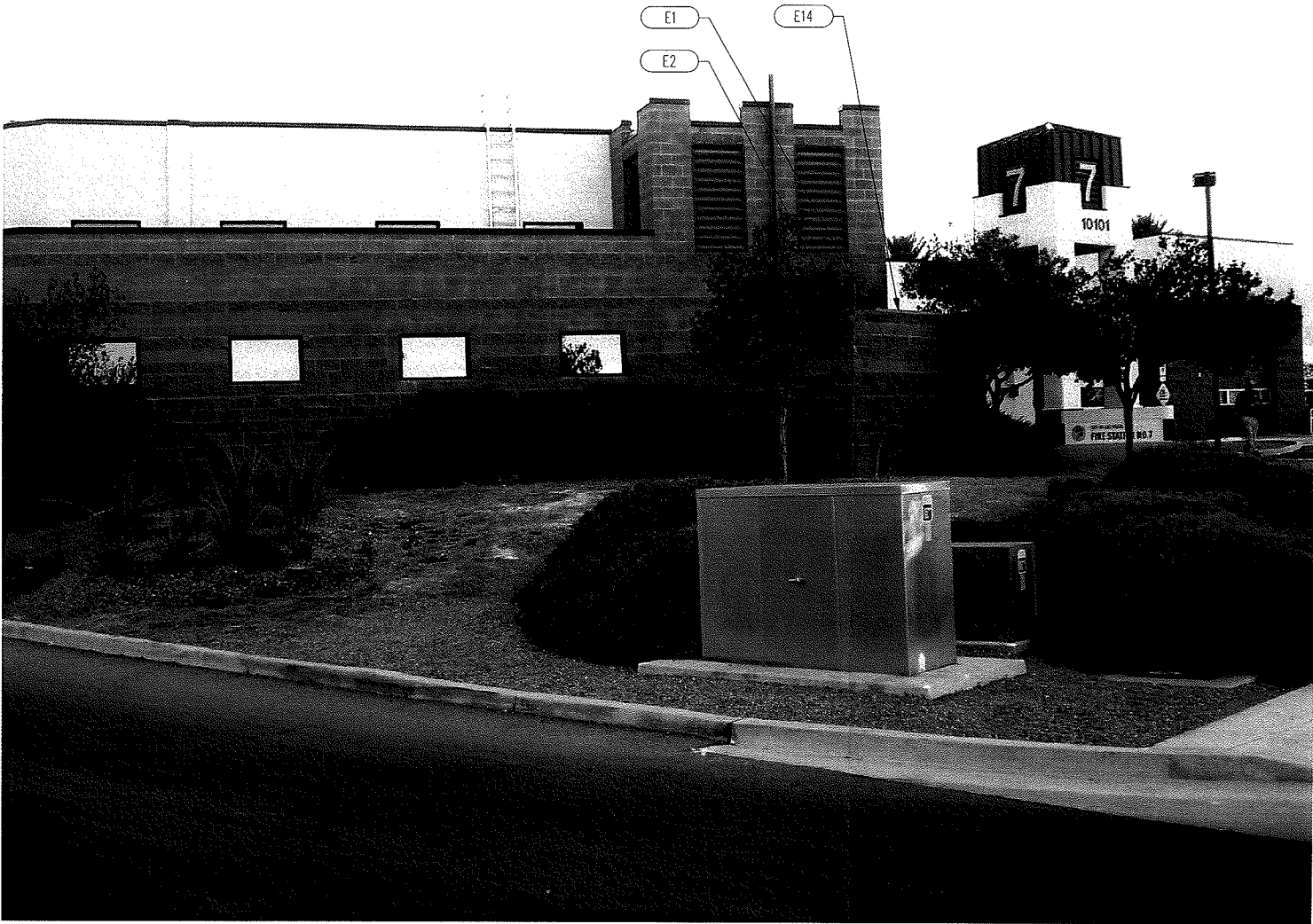
EXISTING BUILDING PHOTO
