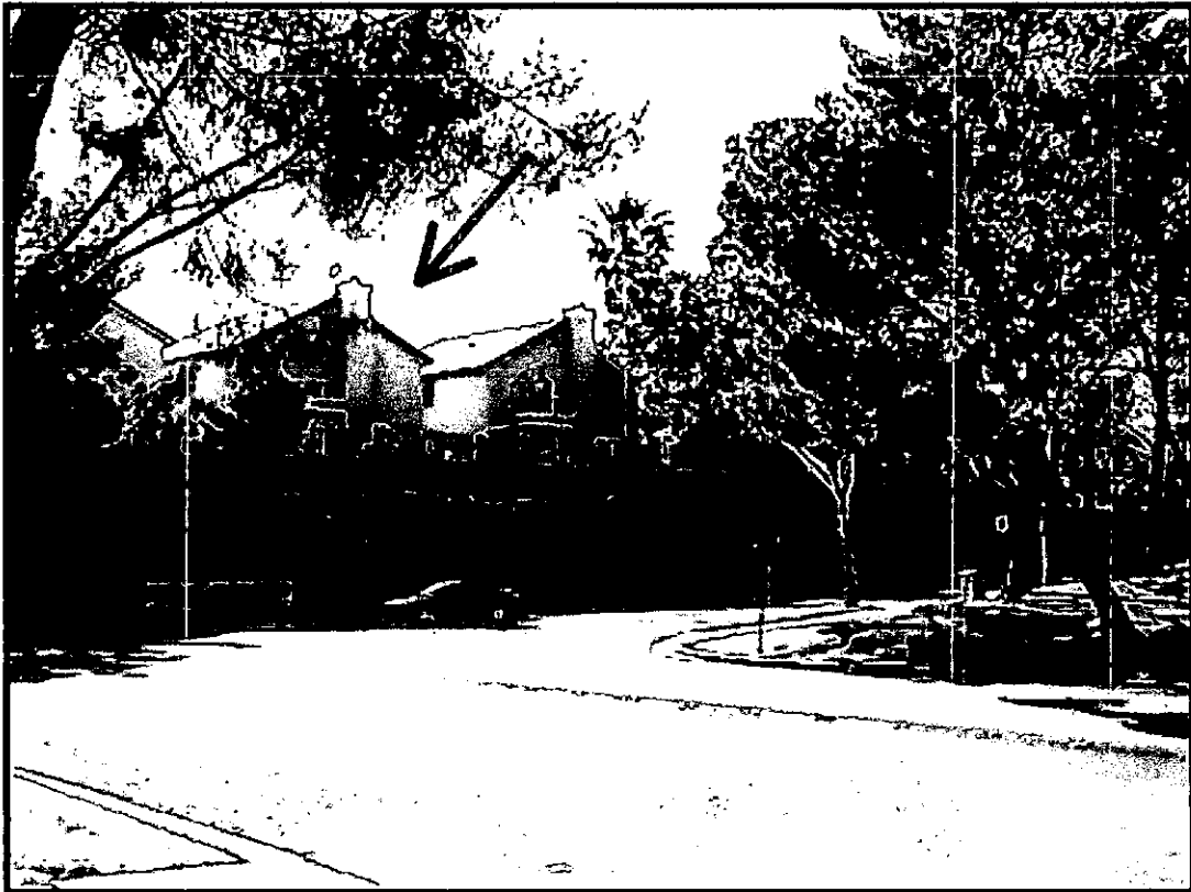
VIEW OF 3016 YANKEE CLIPPER DR. FROM STARBOARD DRIVE
