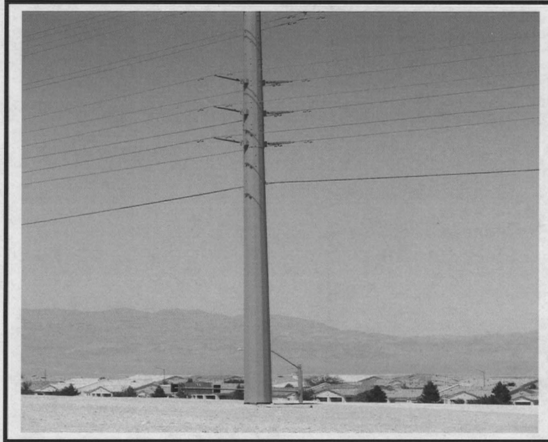
Existing View Looking North East
