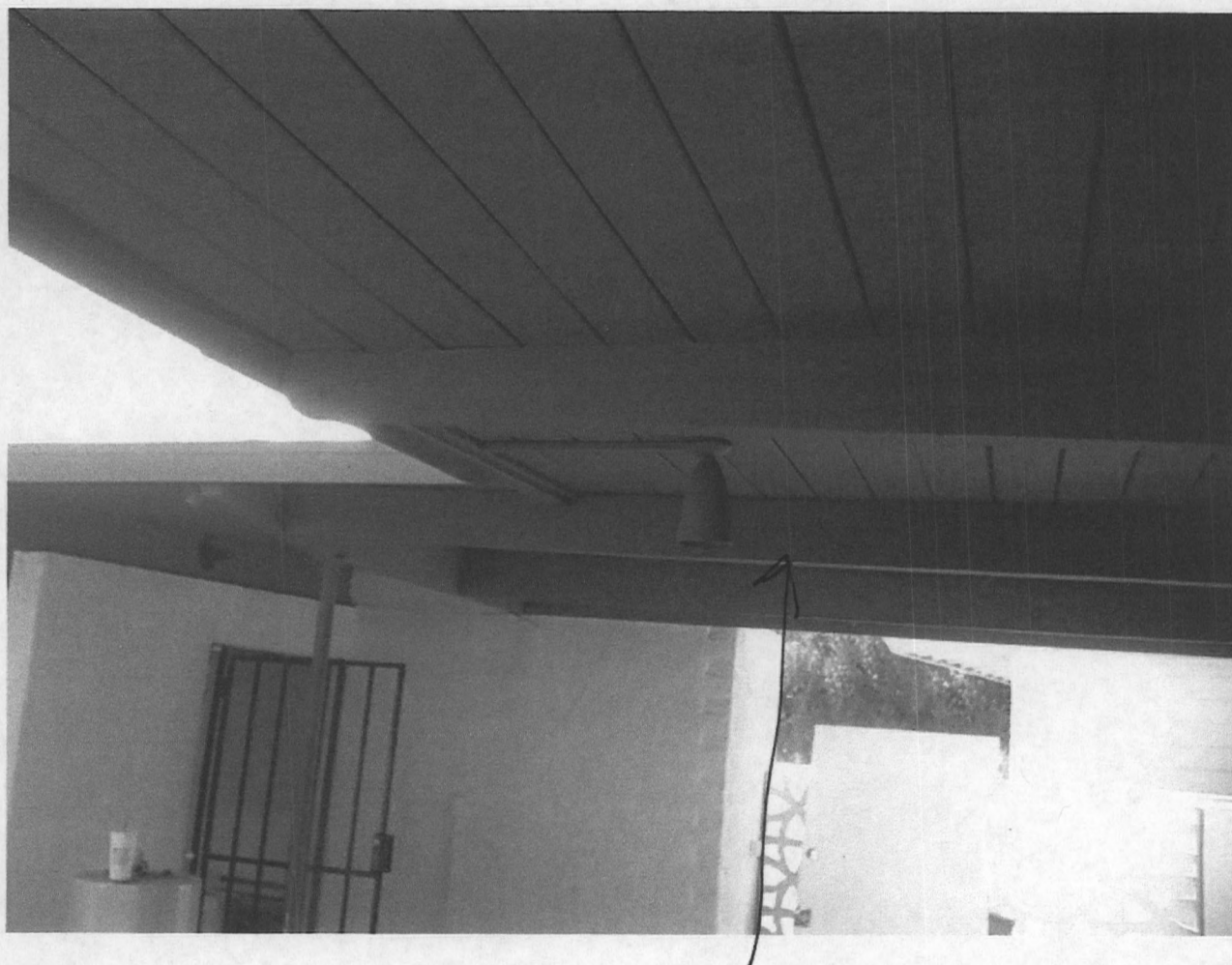
Roof Detail from House
