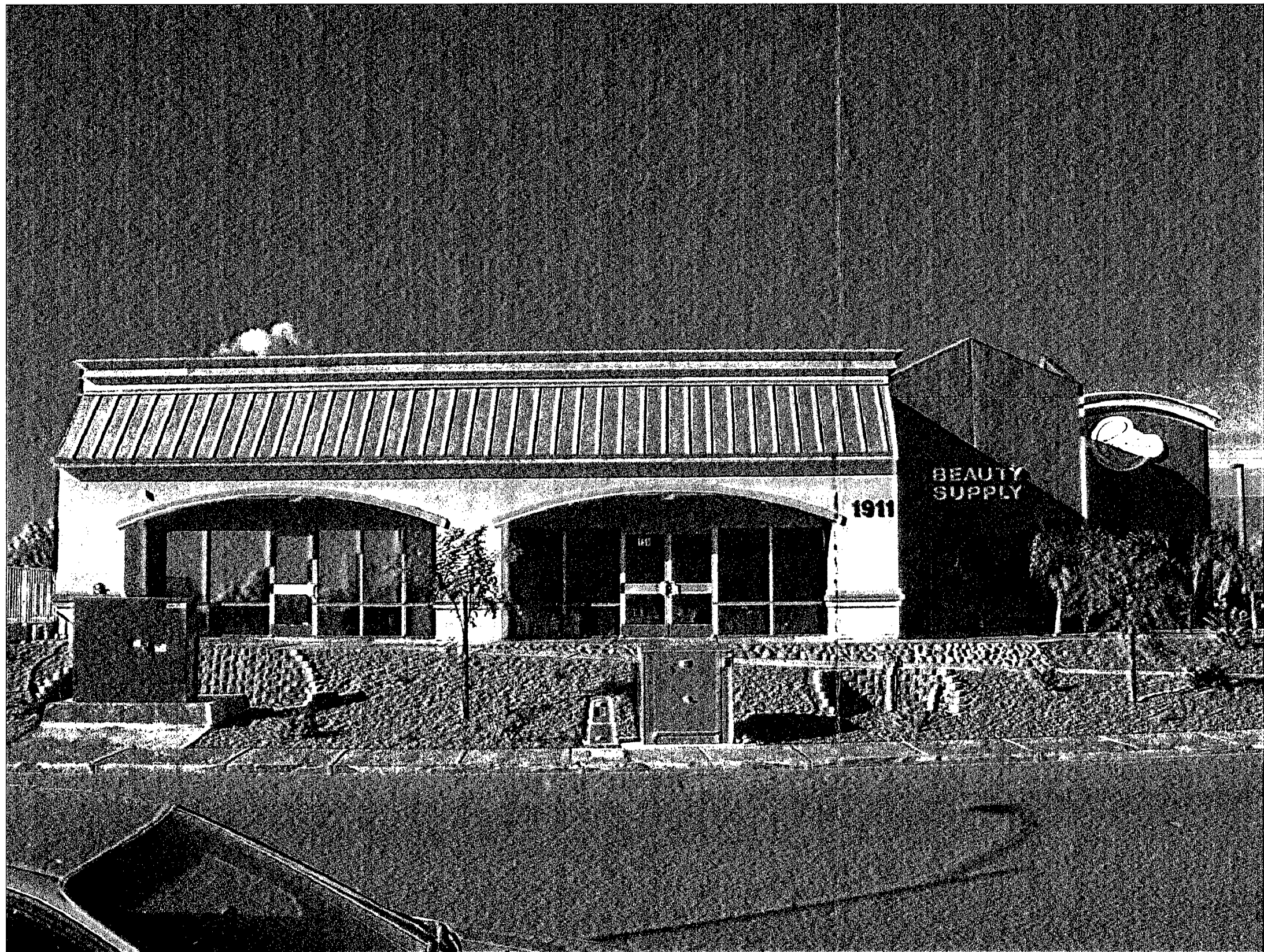
EAST ELEVATION (FUTURE GRITZ CAFE ENTRANCE)
