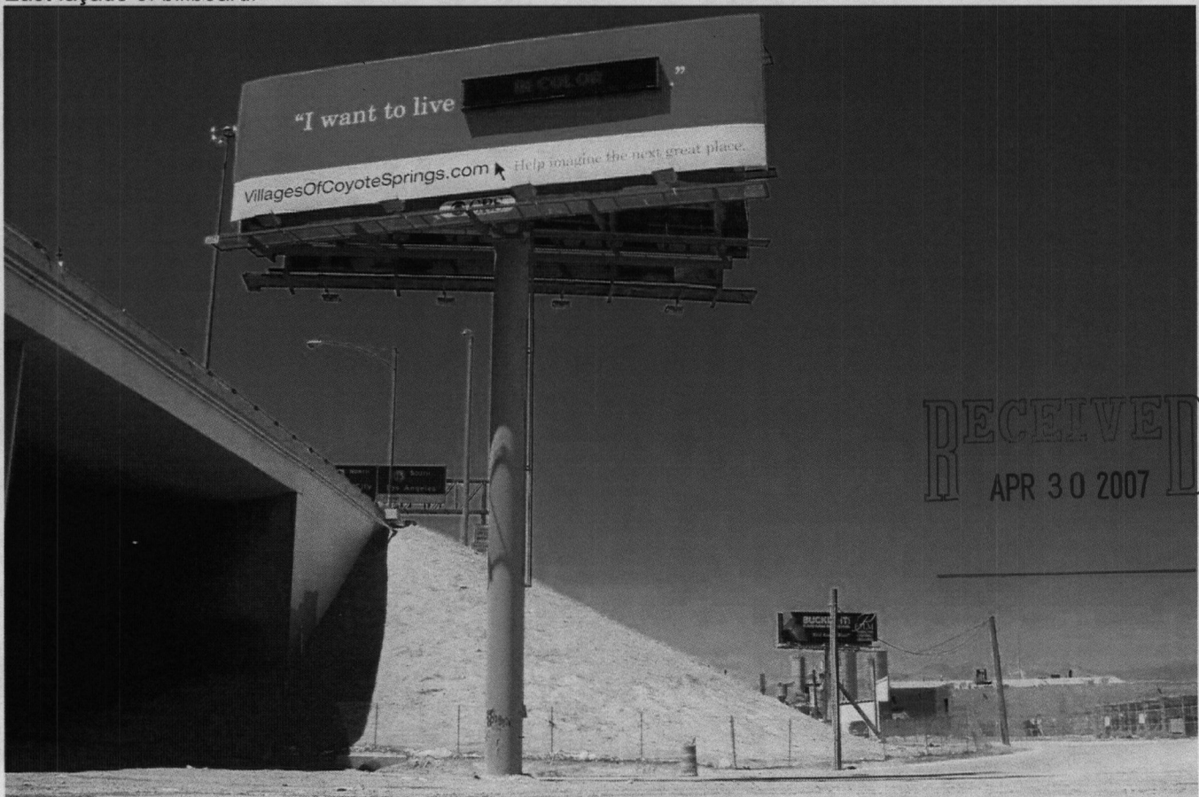
East façade of billboard, full shot. Note graffiti at base of pole.
