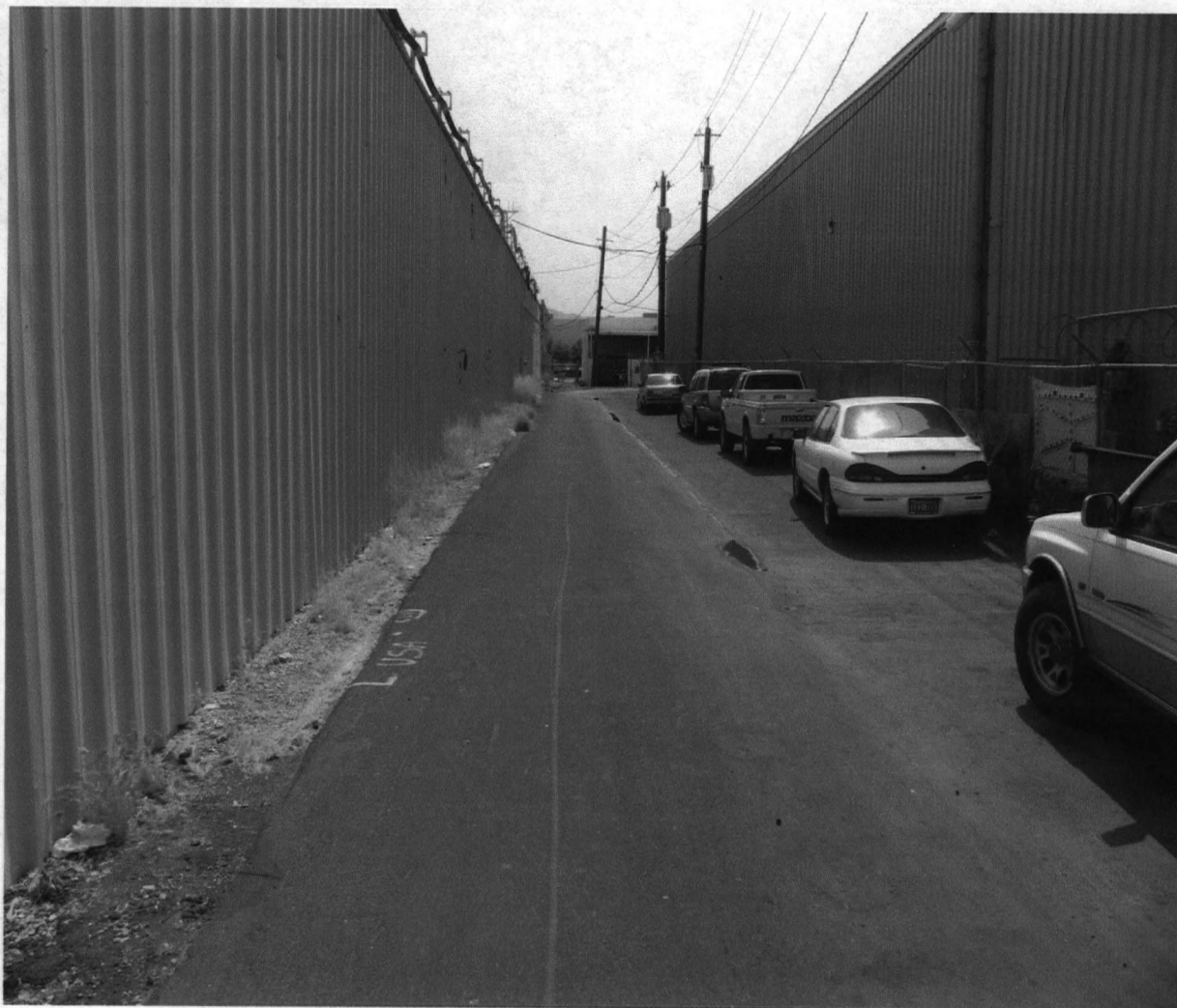
SOUTH BUILDING WALL LOOKING EAST
