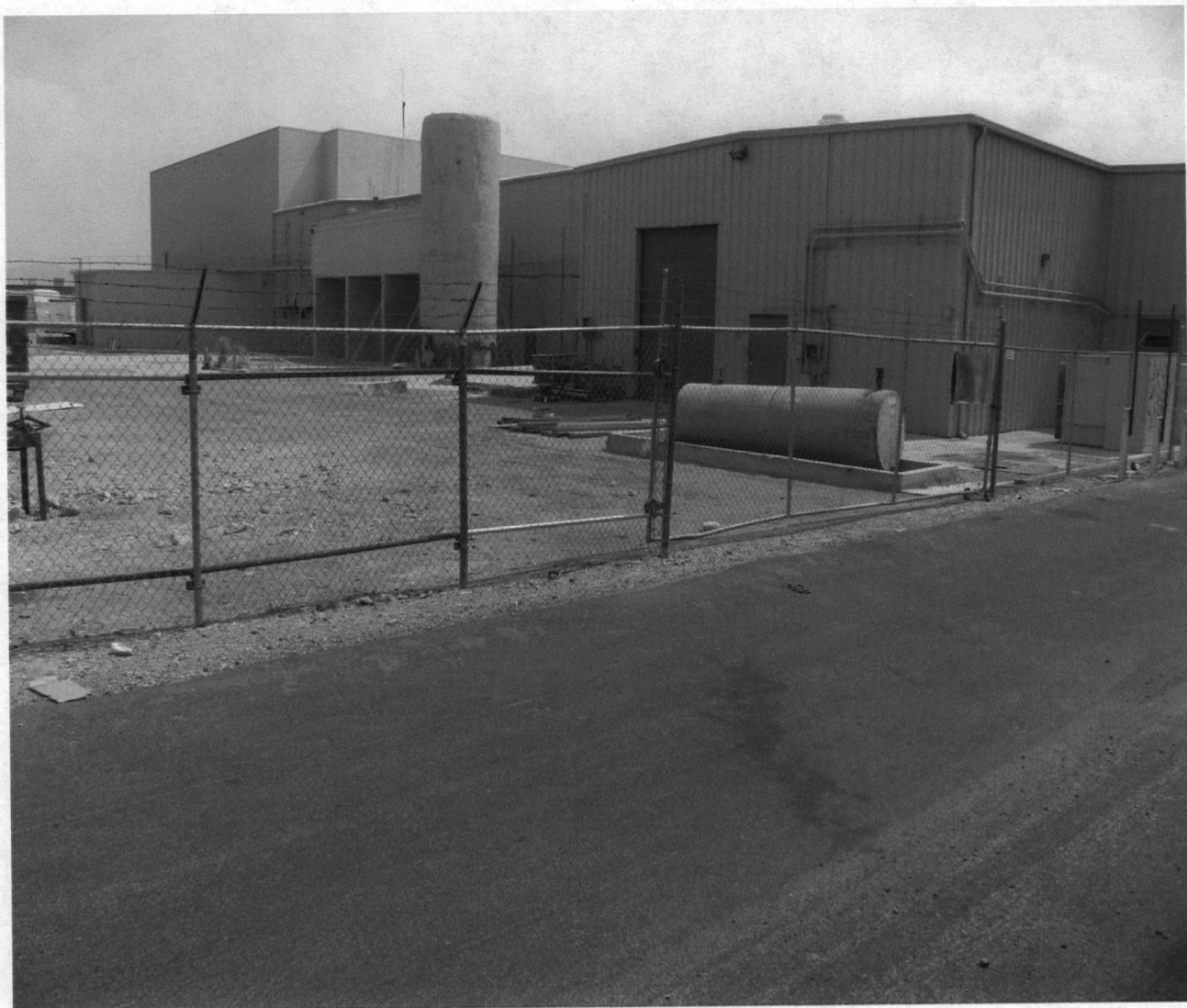
LOOKING NORTHEAST AT BUILDINGS
