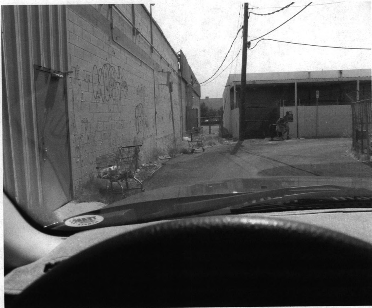
SOUTH BUILDING WALL LOOKING EAST
