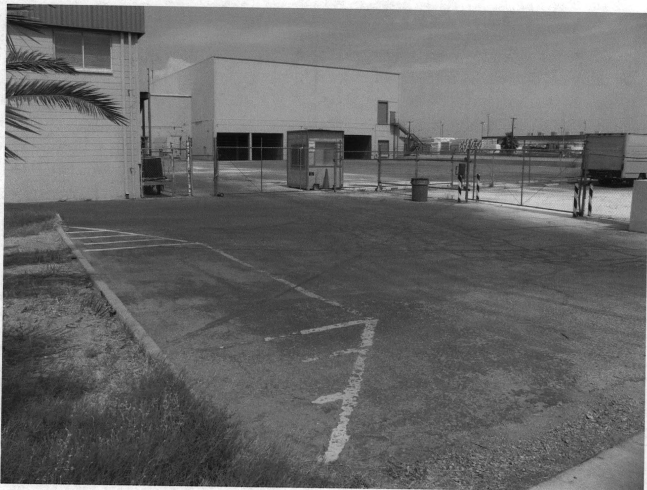
FRONT PARKING AREA LOOKING NORTHWEST FROM MOJAVE
