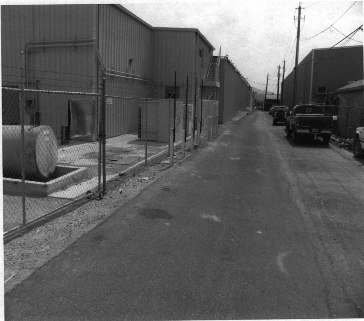
SOUTH PROPERTY LINE LOOKING EAST
