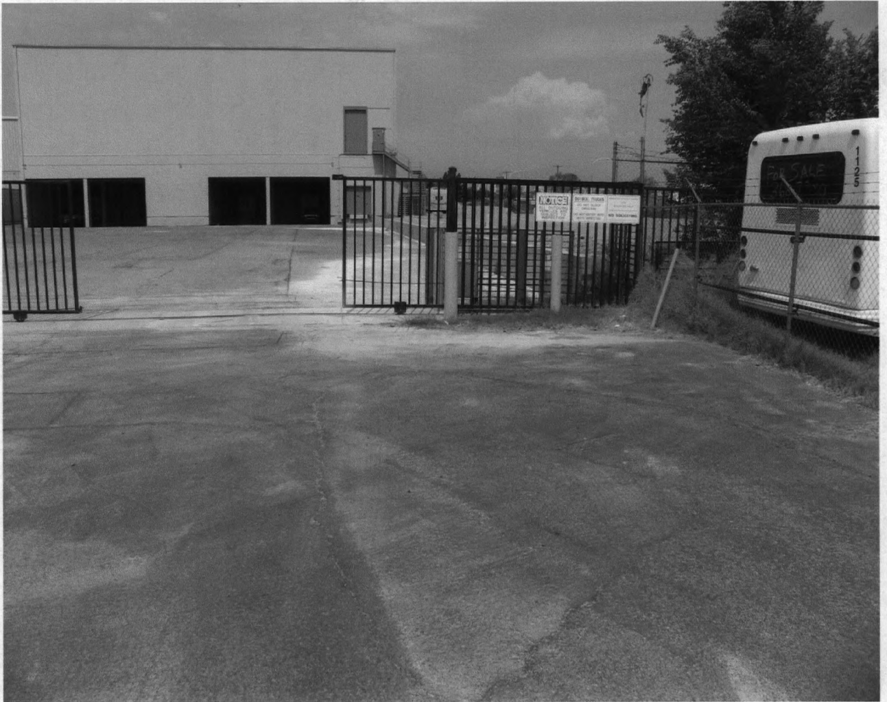
MAIN ENTRANCE LOOKING WEST FROM MOJAVE
