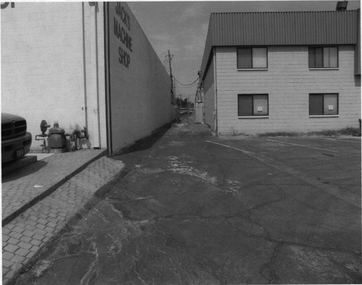
SOUTH PROPERTY LINE LOOKING WEST FROM MOJAVE
