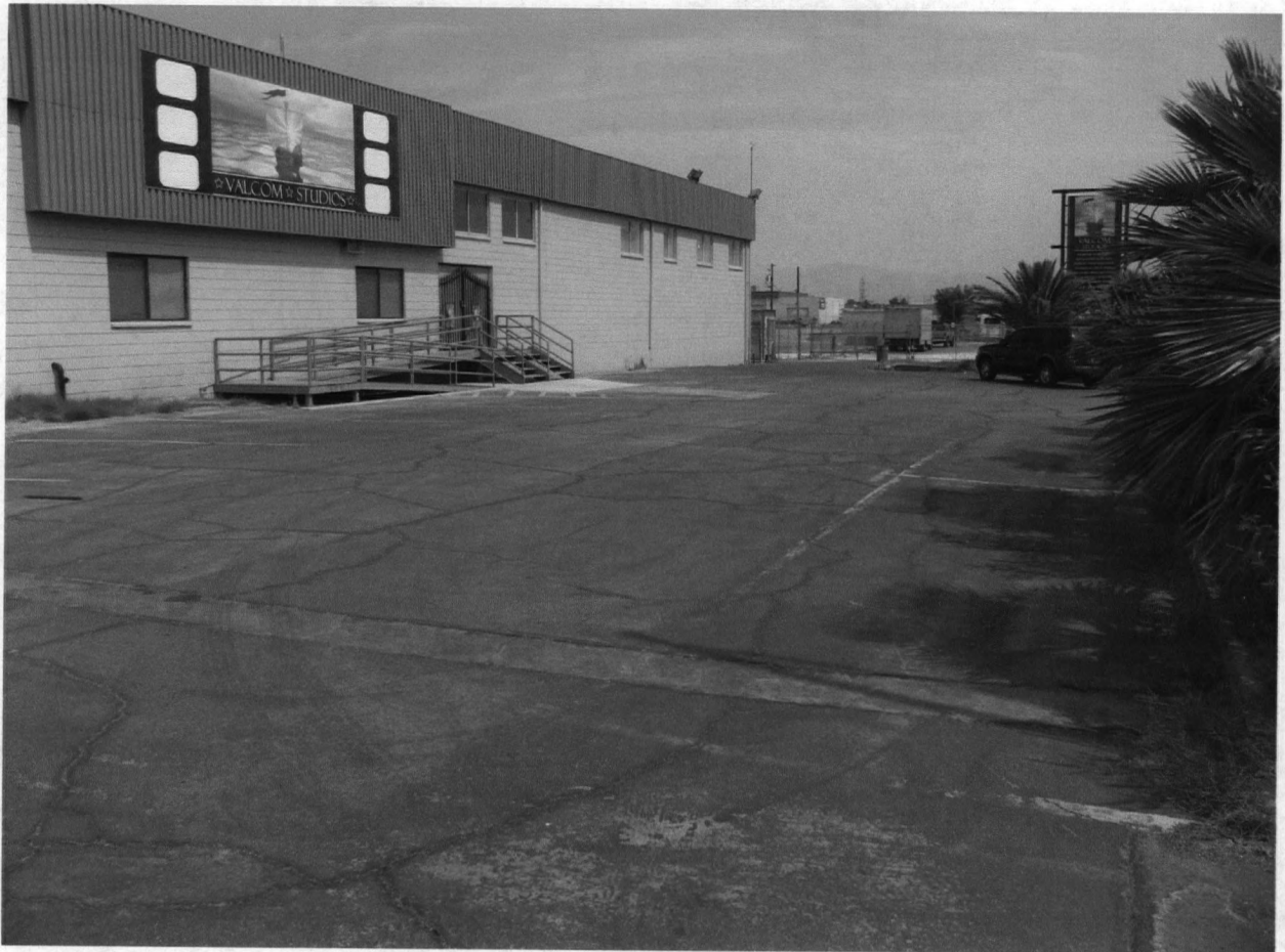
FRONT OF BUILDING AND PARKING LOT FACING MOJAVE LOOKING NORTHWEST
