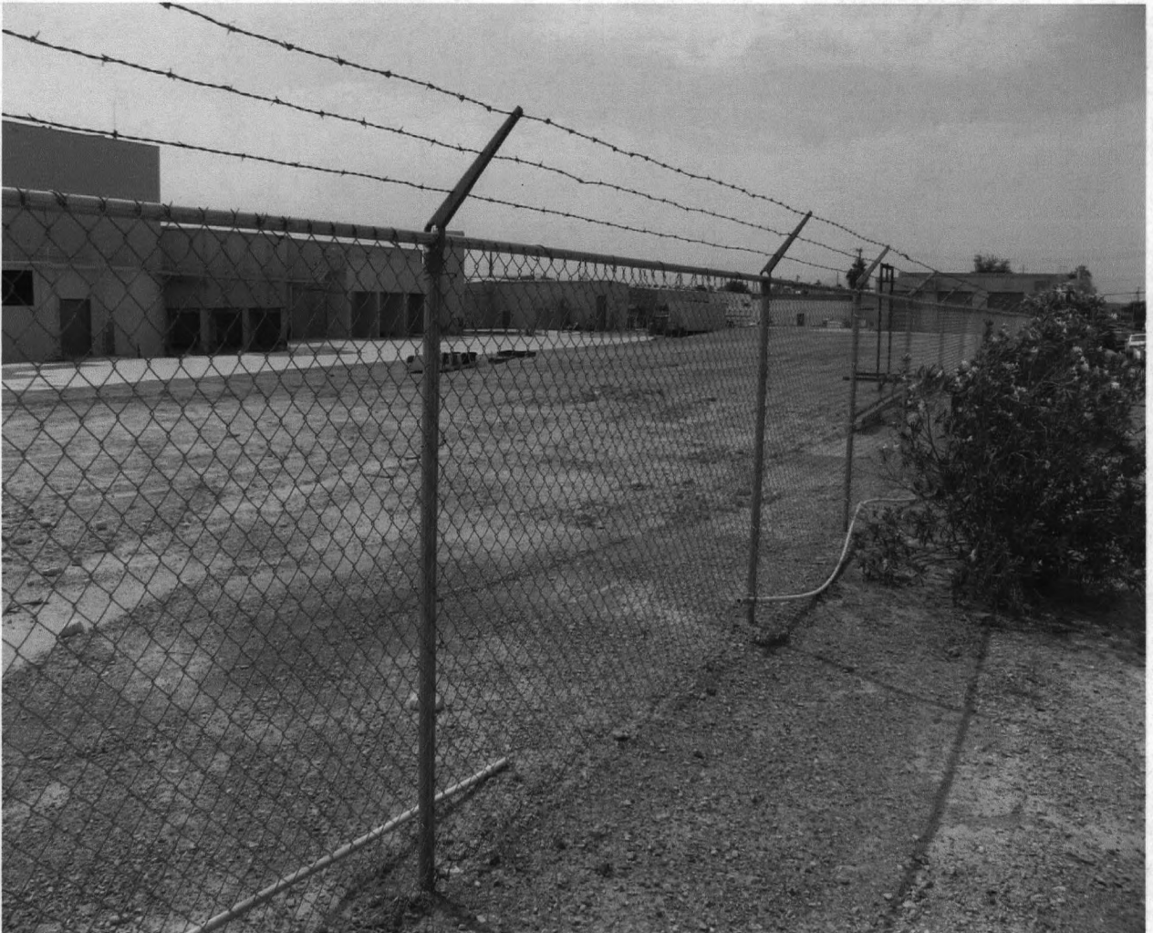
WEST PROPERTY LINE ON 30 TH STREET LOOKING SOUTHEAST AT BUILDING
