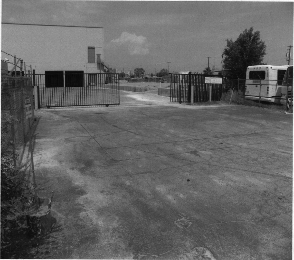
MAIN ENTRANCE LOOKING WEST FROM MOJAVE
