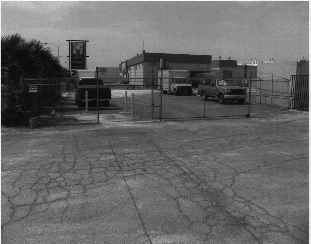
MAIN ENTRANCE LOOKING SOUTH
