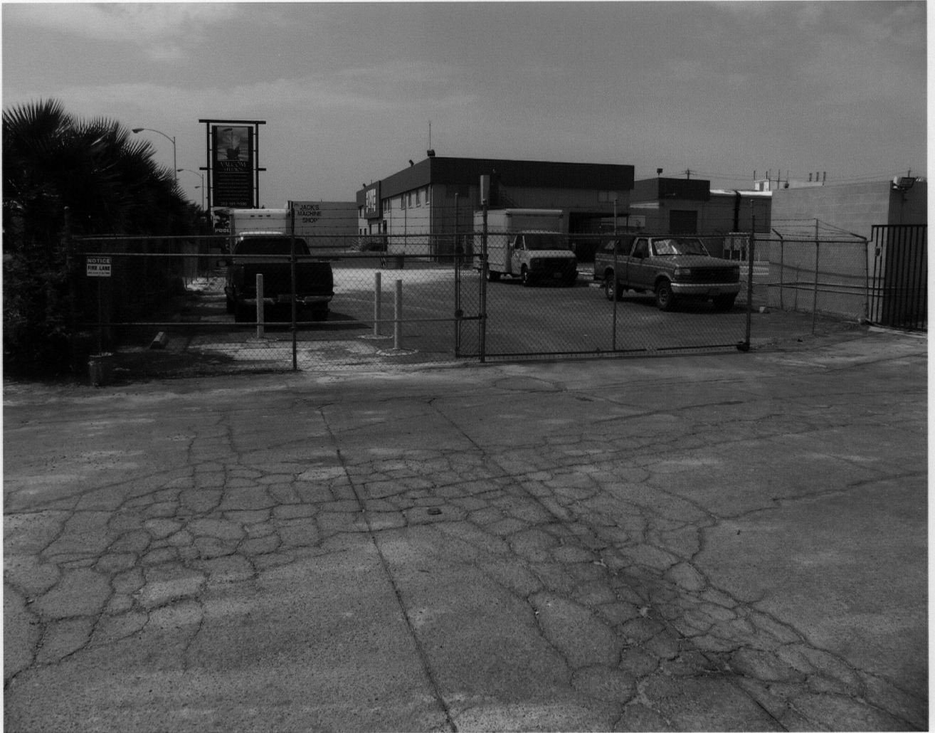
MAIN ENTRANCE LOOKING SOUTH
