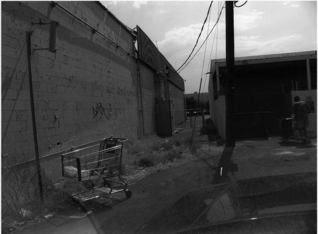
SOUTH BUILDING WALL LOOKING EAST
