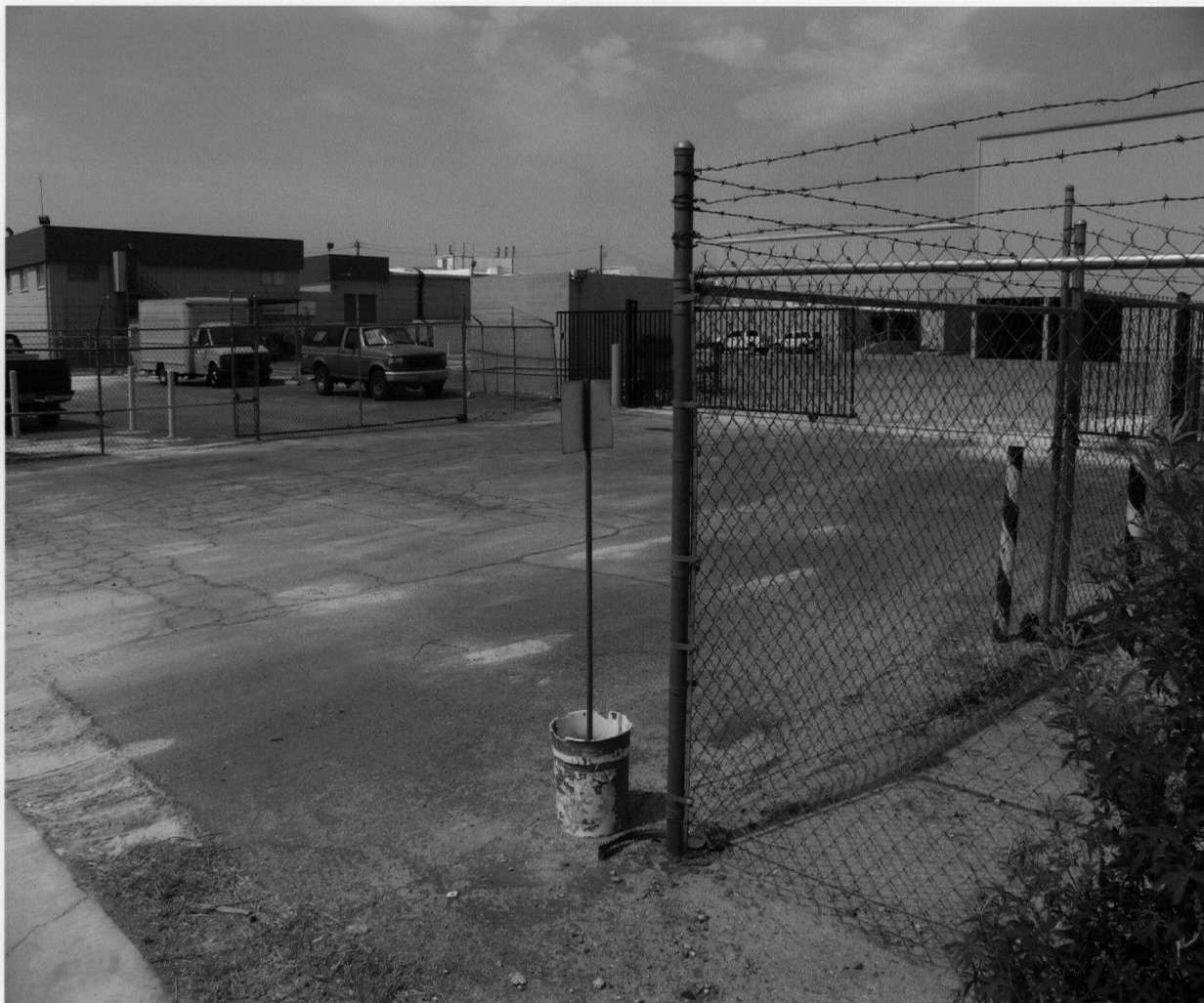
MAIN ENTRANCE OFF MOJAVE LOOKING SOUTHWEST.
