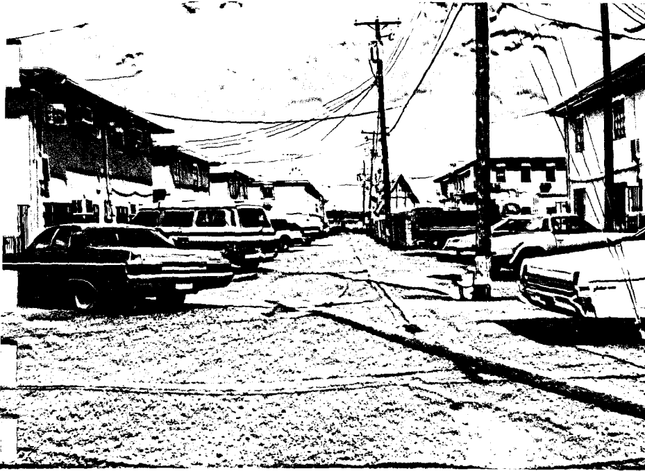
Photograph shows rear of subject buildings and the alleyway which is assumed to be abandoned.
