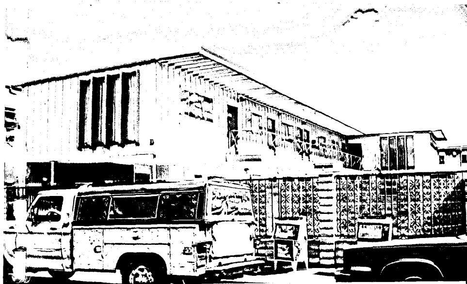
Looking southeasterly at the third Meadows building located on Baltimore.
