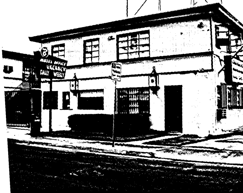
Looking northwesterly at the Biltmore Motel.
