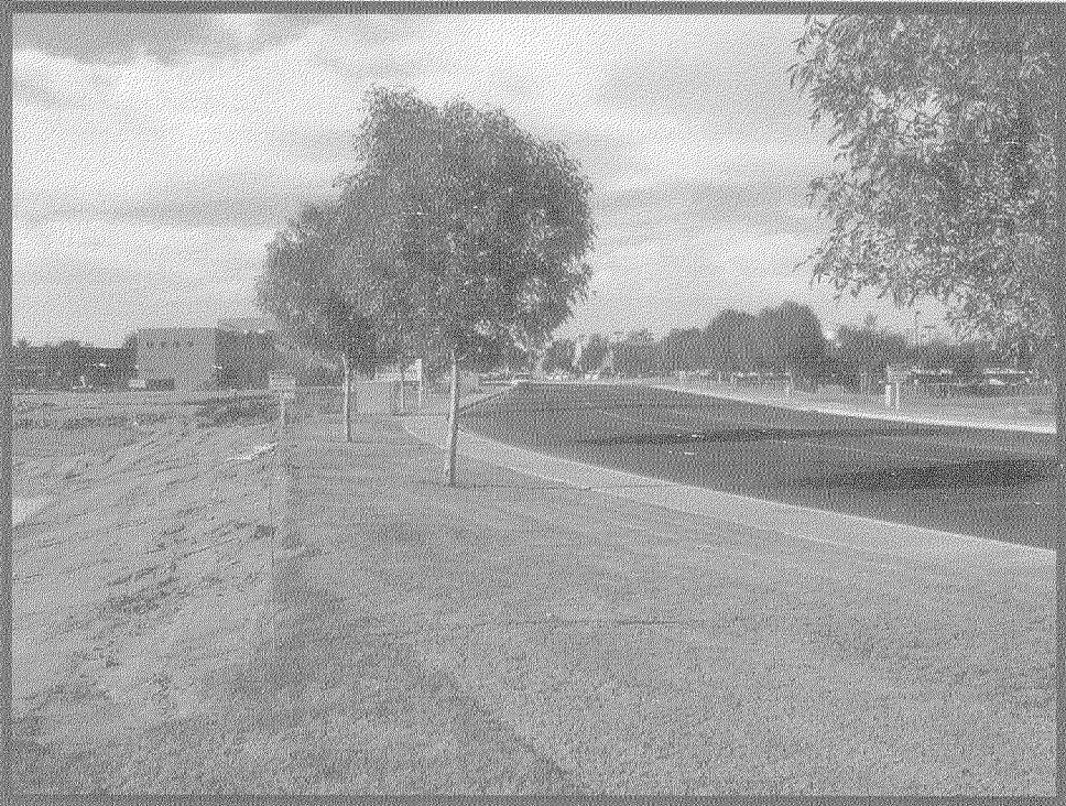
Flagging and wooden stakes help to protect existing trees and groundcover (Courtesy of Maricopa County)
